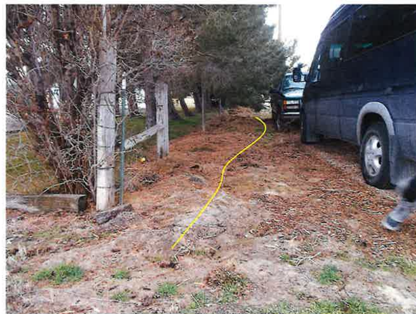
Buried Pipe running south along fence to valve box
