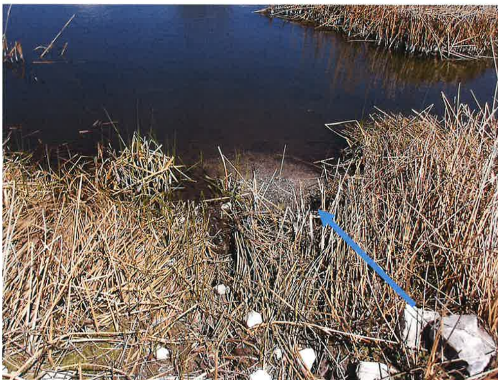
Flow of water into reservoir from pipeline (obscured by rocks and cattails). Arrow shows direction of flow. Note gravel deposit created by inflow.
