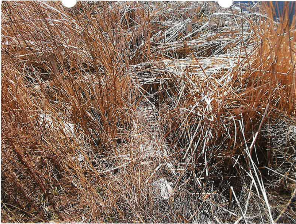
Spillway of dam partially obscured by cattails.
