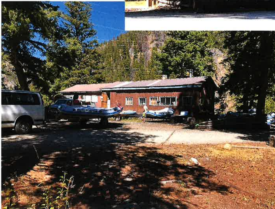
Boat Wash Station
