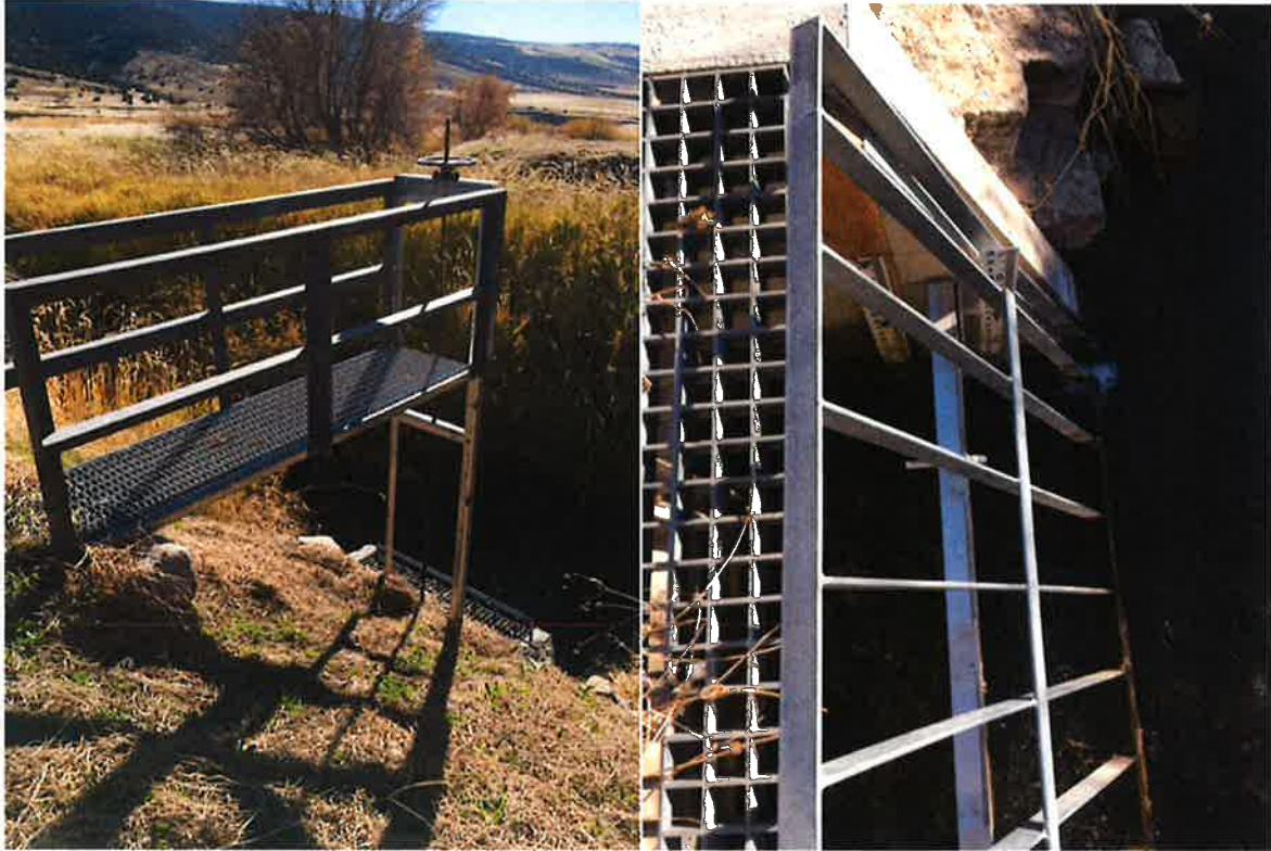
Point of Diversion & Measuring Device
