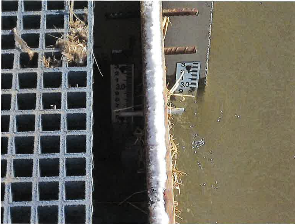
Above: Upstream and downstream staff gages at POD. Below: Place of use (upper pond)
