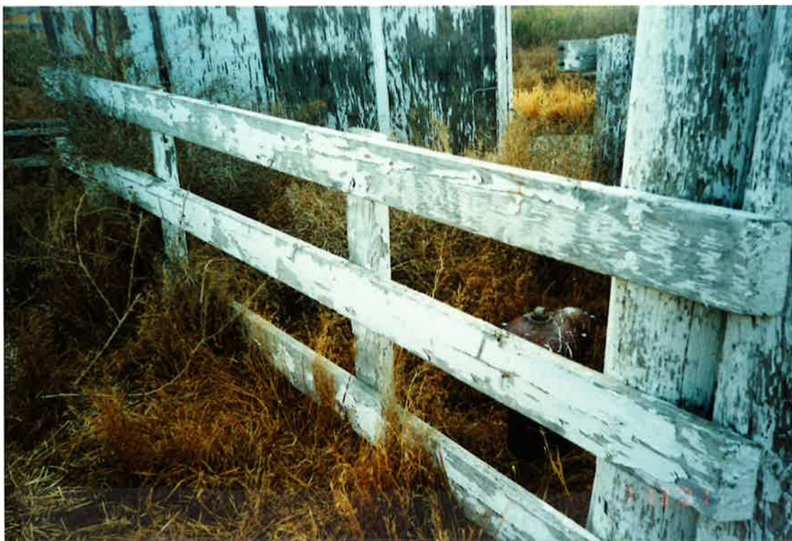
Well #2 (looking SE)
