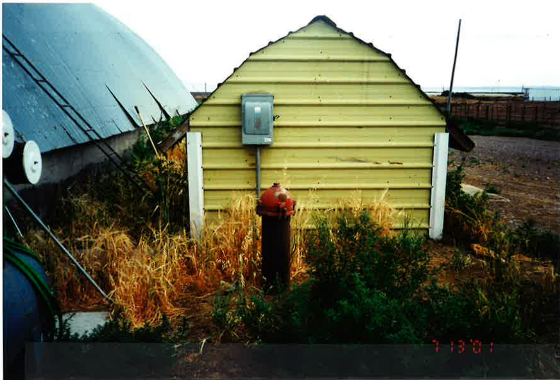
Well #1, Well House (Looking North)
