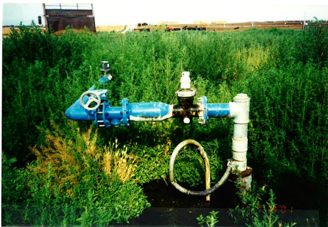
Well & Mainline for Dust Control (Looking West)
