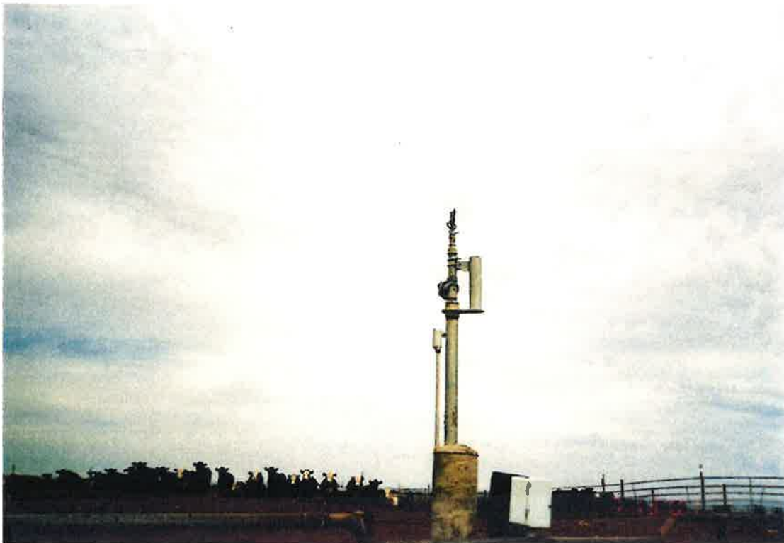
Figure #2: A sprinkler on the dust abatement system
