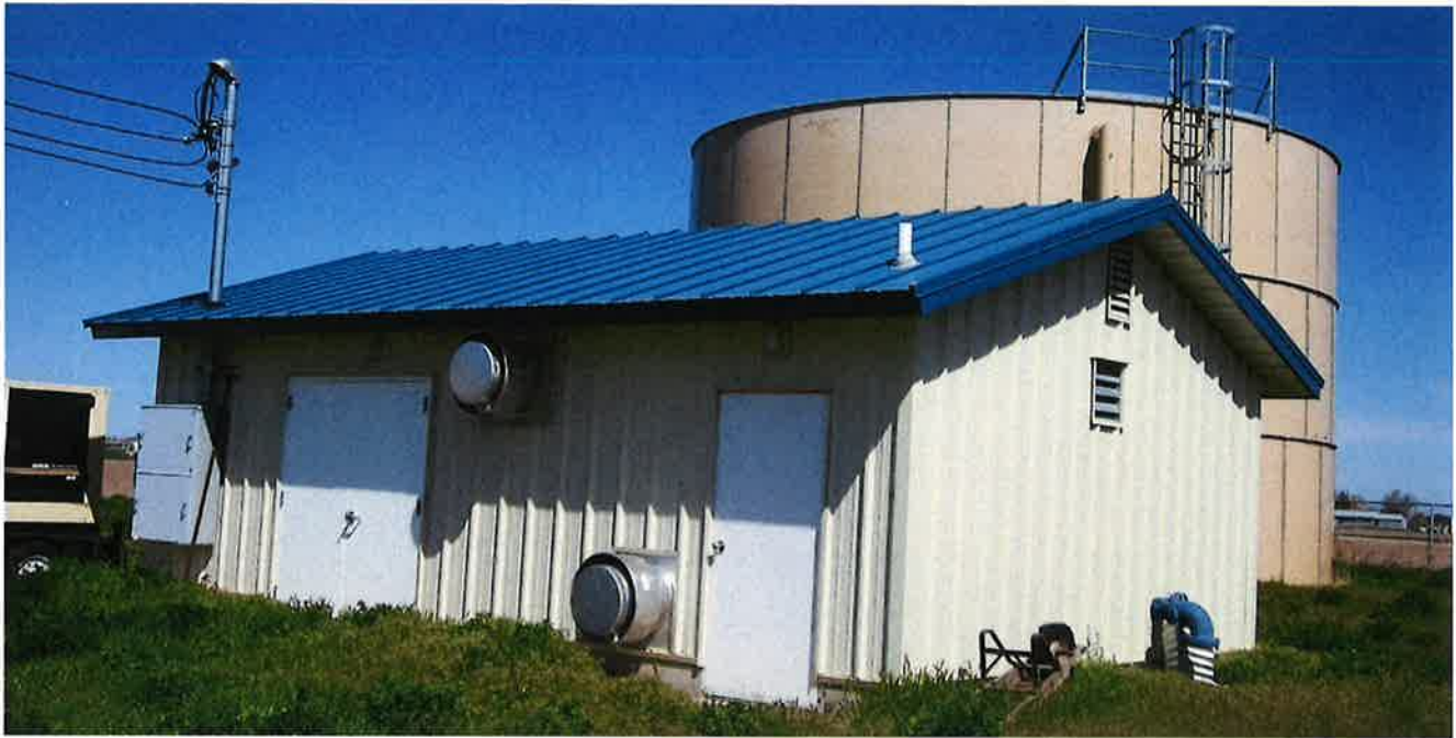
Above: New well pump house and water tank.
