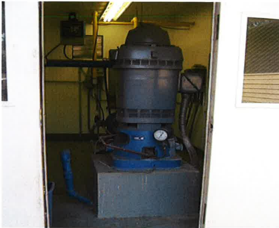
Above: New well motor and pump
