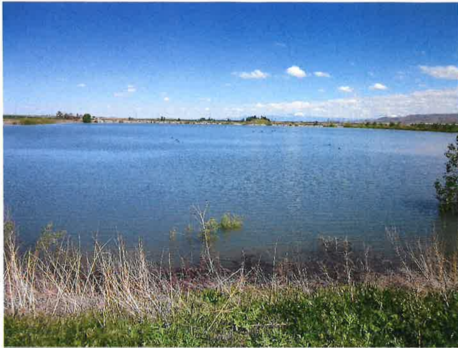
Figure 1: Looking east across east reservoir
