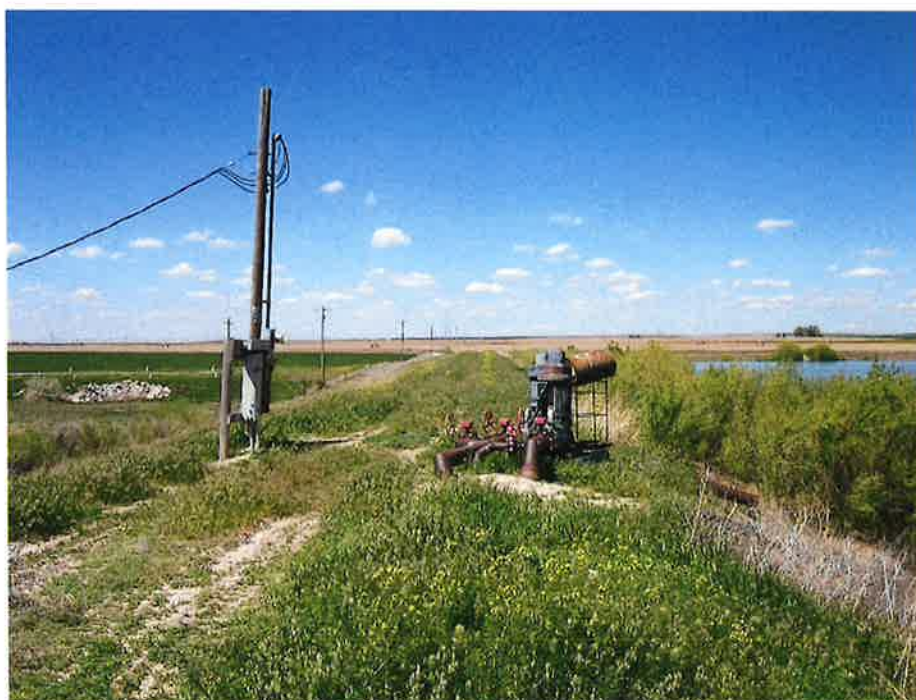
Figure 4: West reservoir pumping station
