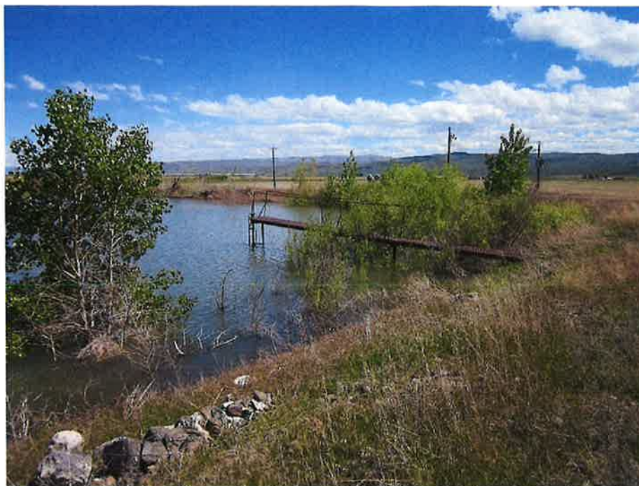
Figure 3: Catwalk and gate to pumping station
