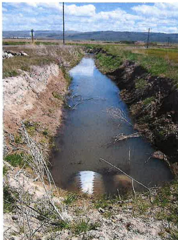
Figure 6: Lower end of ditch at east reservoir
