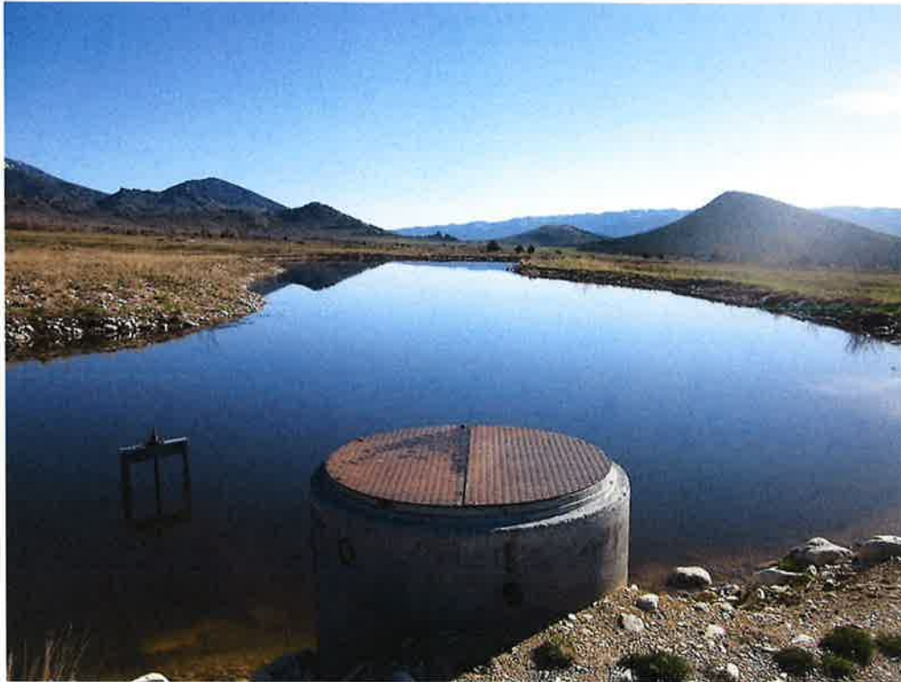
Figure 3: Water control structure at south end of pond
