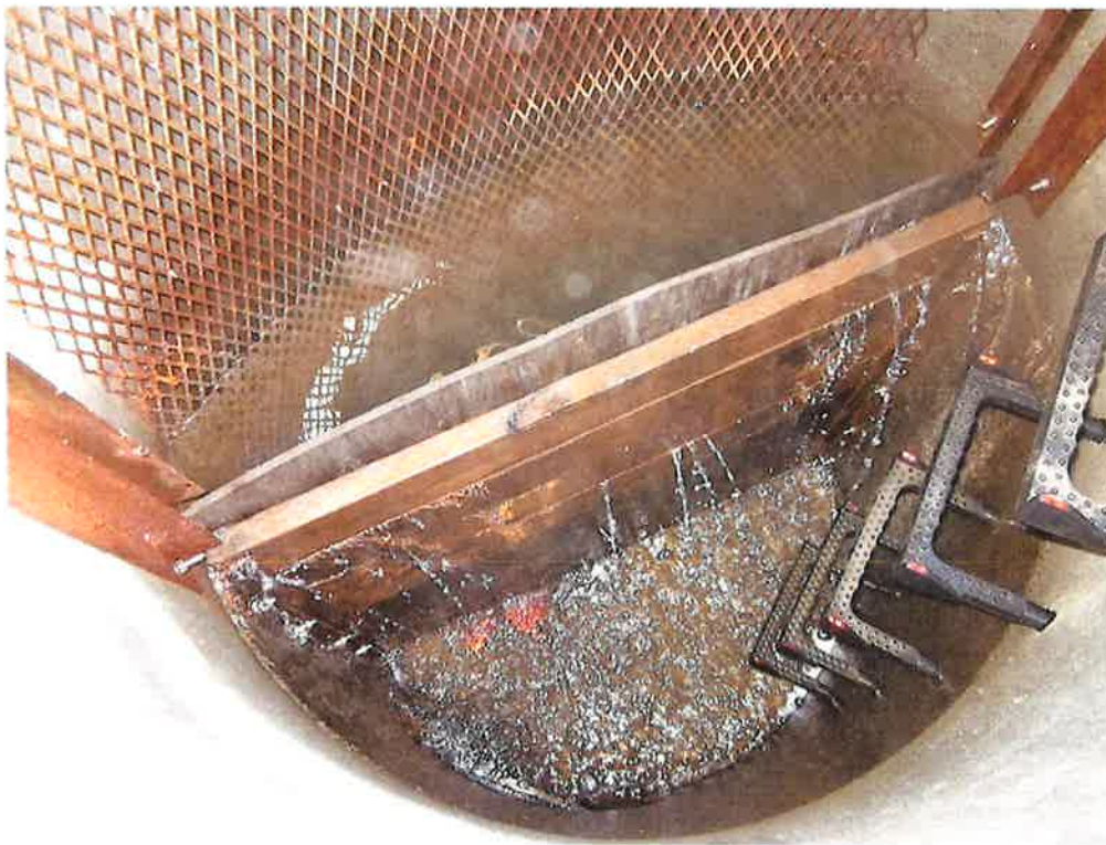
Figure 4: Inside the water control structure
