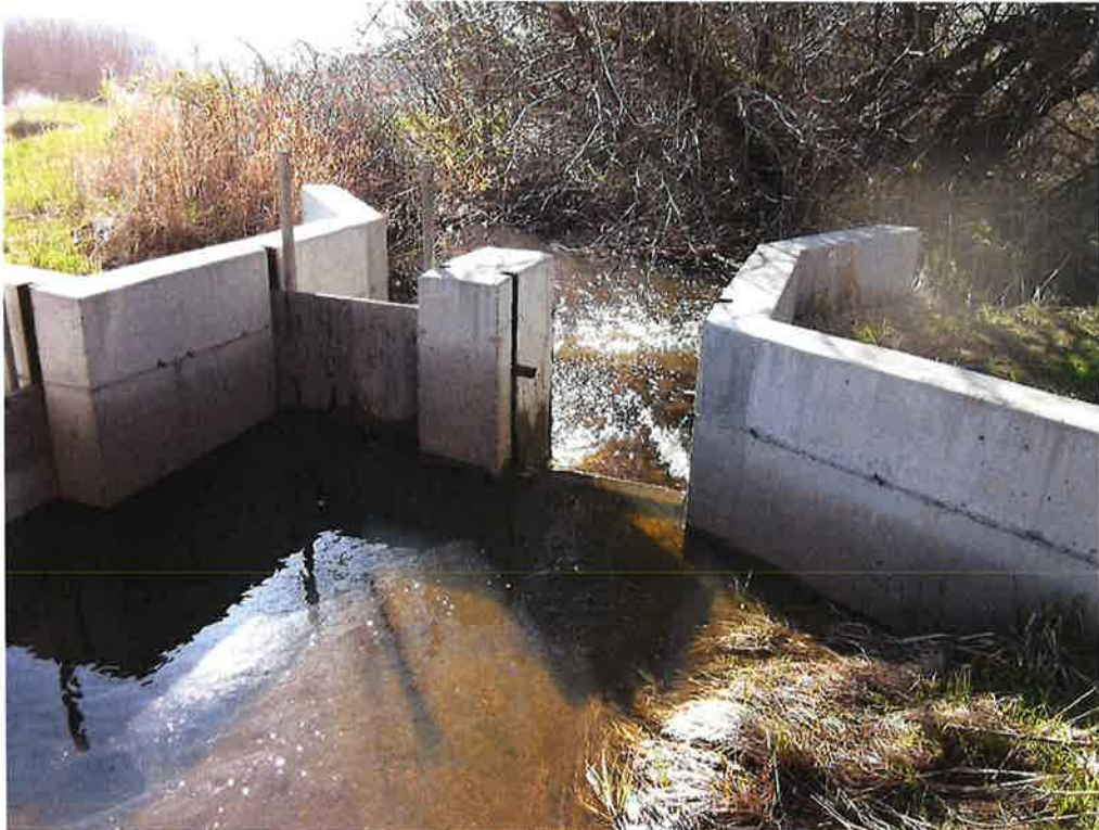
Figure 6: Diversion structure on Almo Creek
