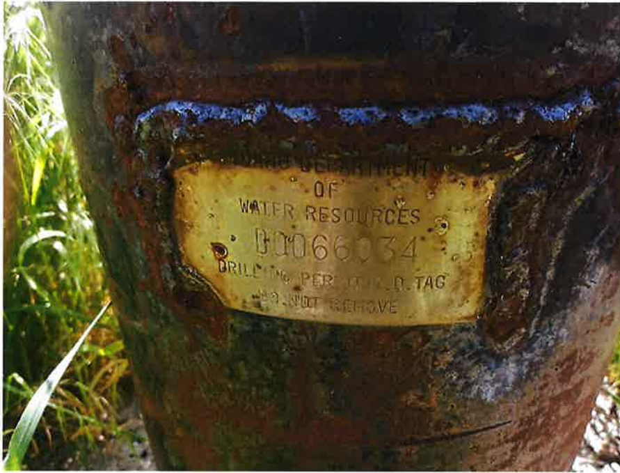
The metal tag welded to the casing of the well. Tag no. D006034
