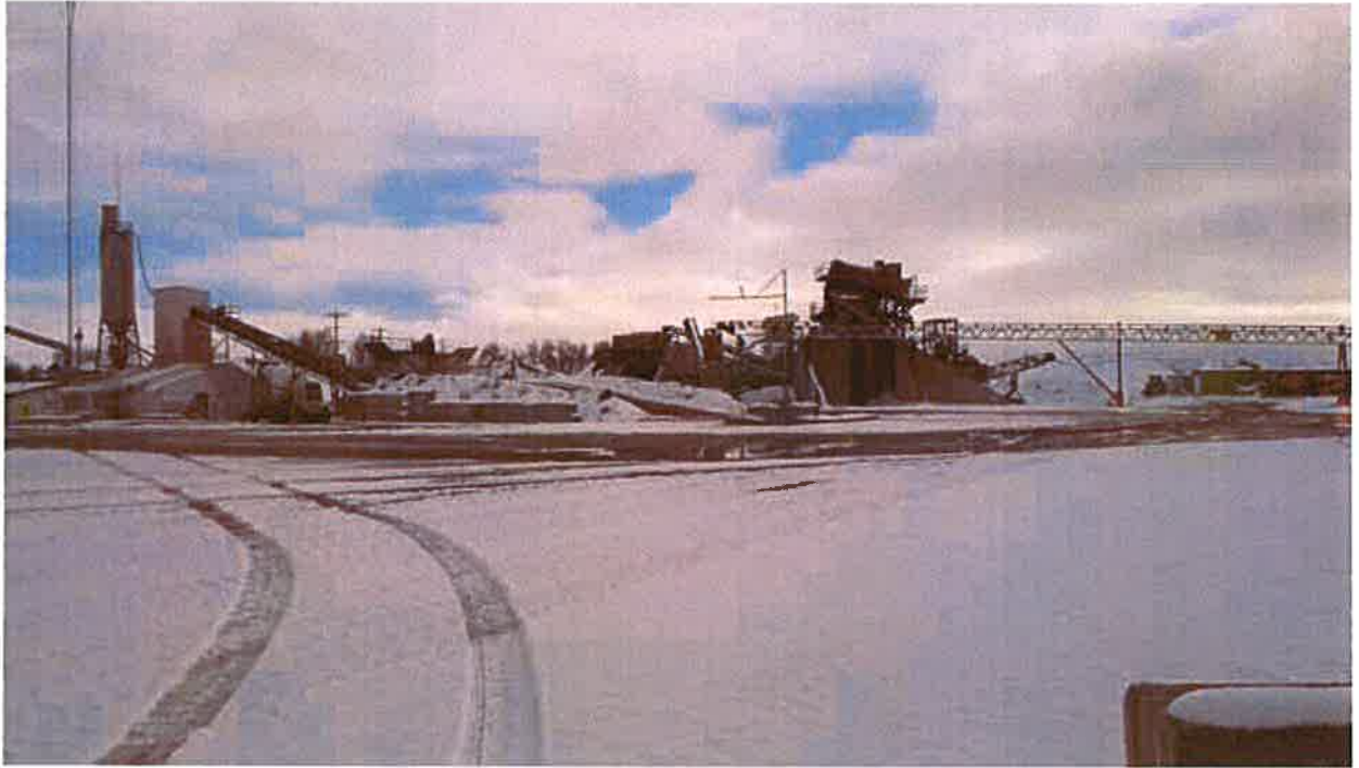
Processing facilities from afar
