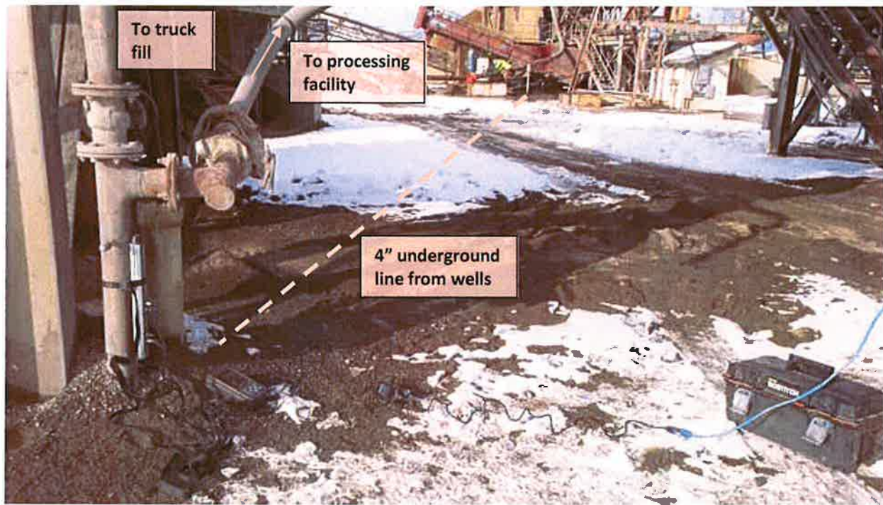
4" line measuring point (crusher wells in background)
