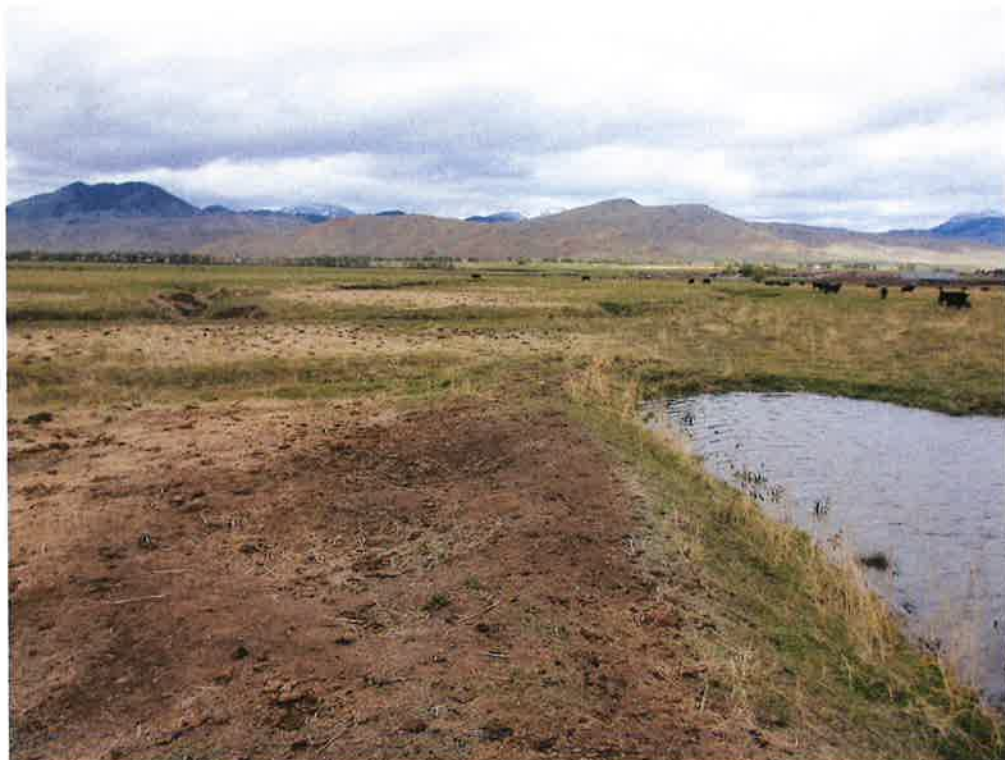
Backup spillway on right abutment of embankment.
