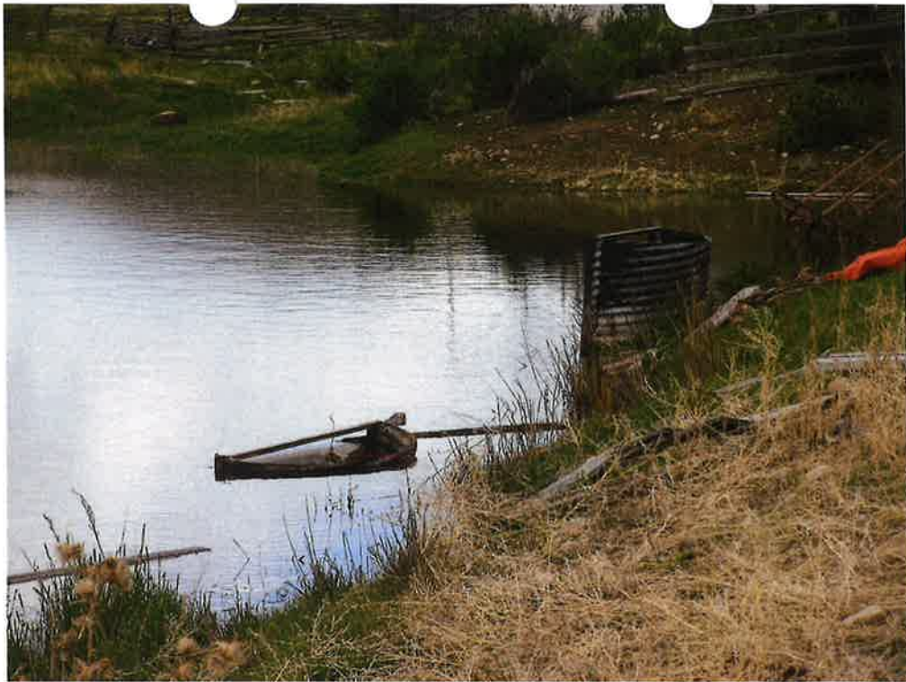
Main spillway (center left) and irrigation headgate (center right).
