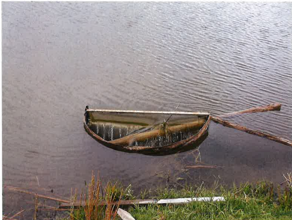
Close-up of main spillway.
