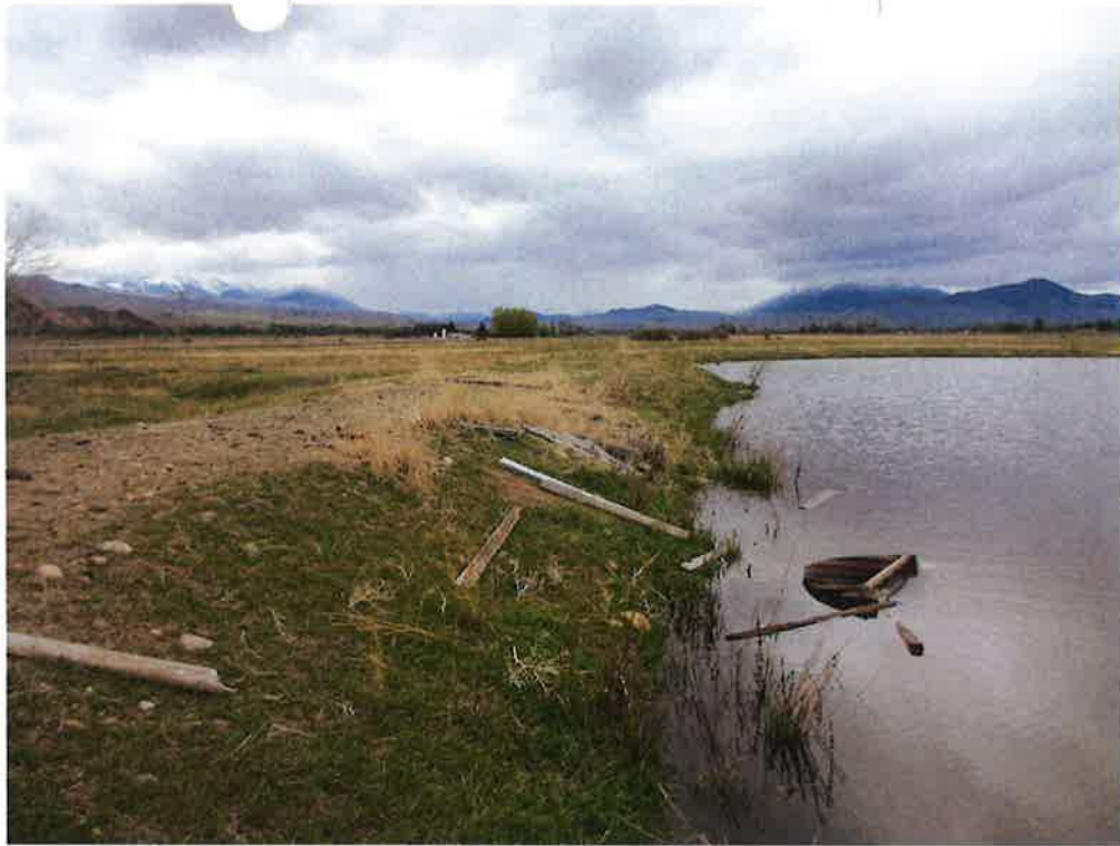
Reservoir embankment with main spillway at right of photo.
