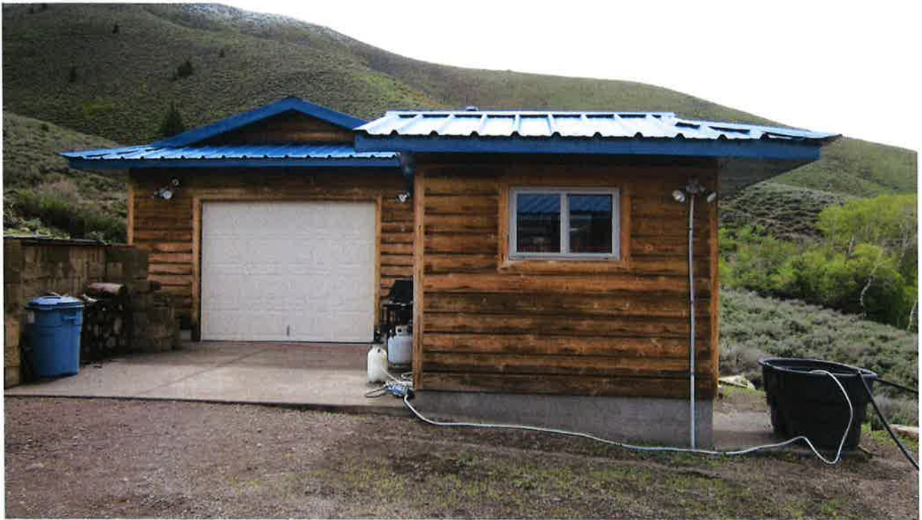
Above: Garage, Seating and Dining Area and a Portable Trough
