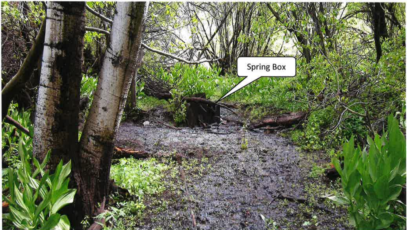
Above: Spring #3, Point of Diversion/Spring Box
