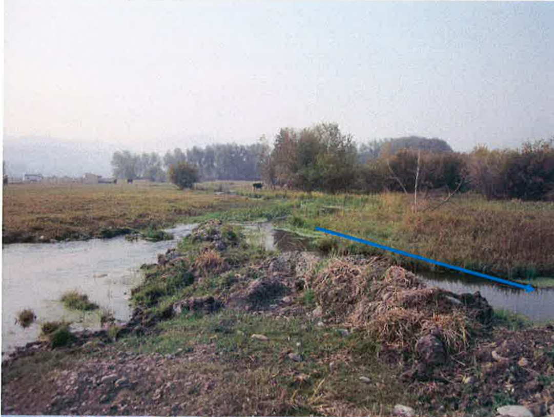
S16 diversion looking upstream
