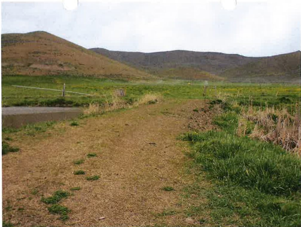
The point of diversion, the Bashaw reservoir embankment.
