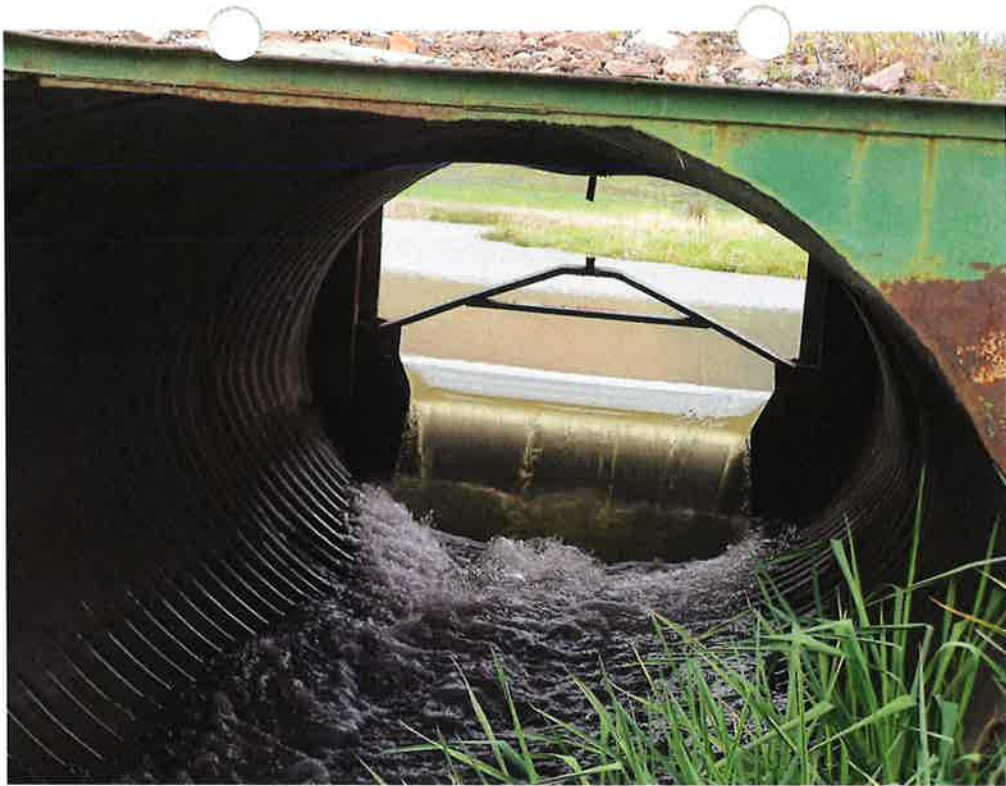
Cipoletti weir at the head of the culvert under the embankment.
