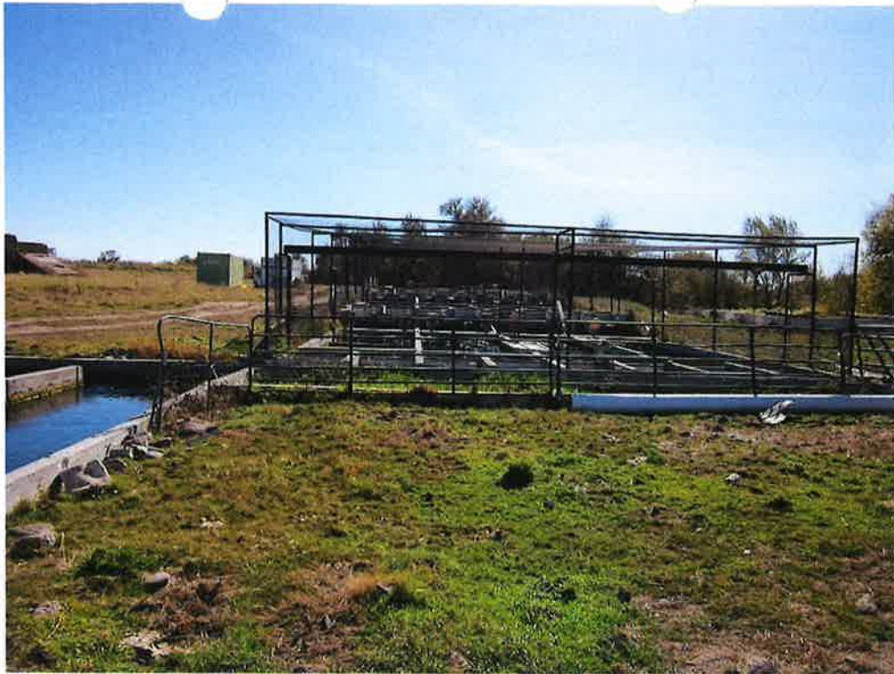
View of South raceways looking south
