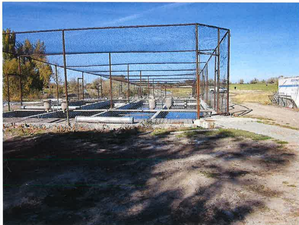
View of South raceways looking north
