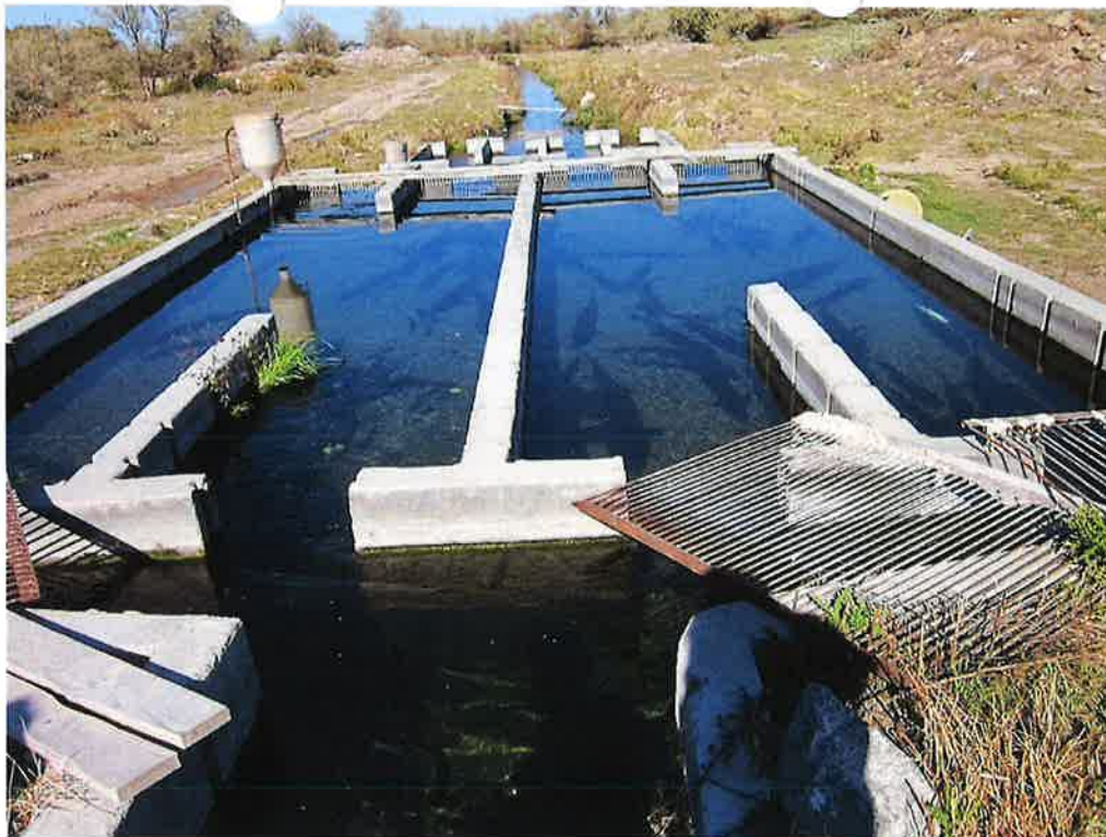
Middle raceways looking north (note sturgeon in raceways)
