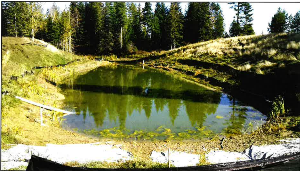
Figure 2: Pond as seen standing on the dam crest facing upstream.
