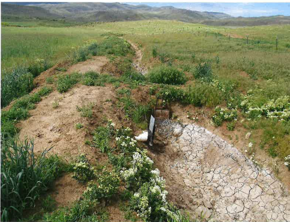
Figure 3. Field headgate as it leads through berm and into gated pipe.
