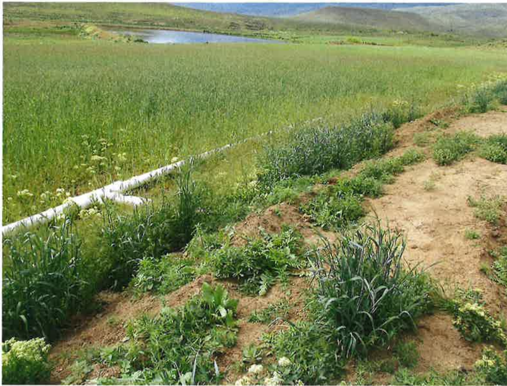
Figure 4. Outlet of field headgate leading into gated pipe along 5.9 acre place of use.
