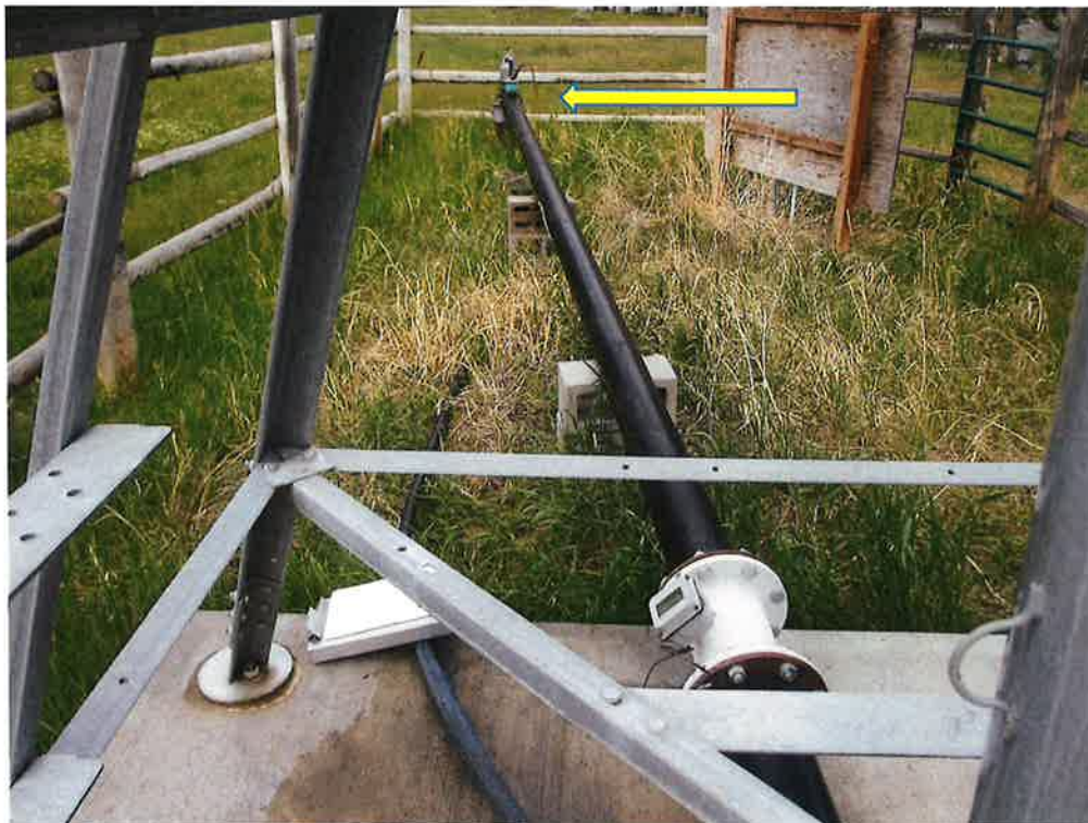
Flow meter installation (well at arrow).
