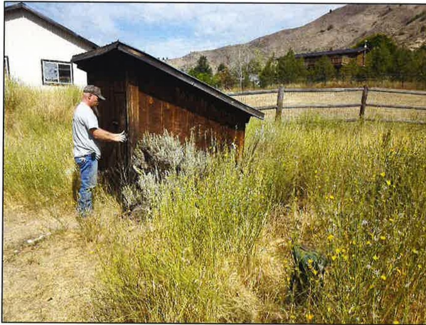
Figure 1: Well 2 pumphouse with well in foreground.
