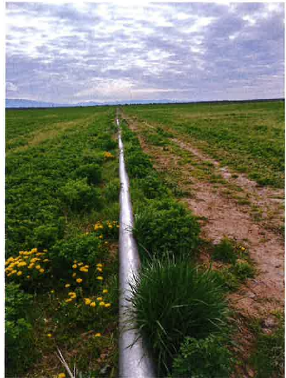
An exposed section of 8-inch pipe between risers
