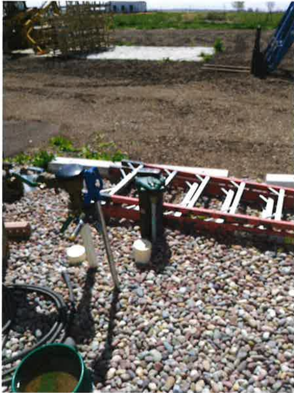
Figure 1 The well head located just south of the production barn.
