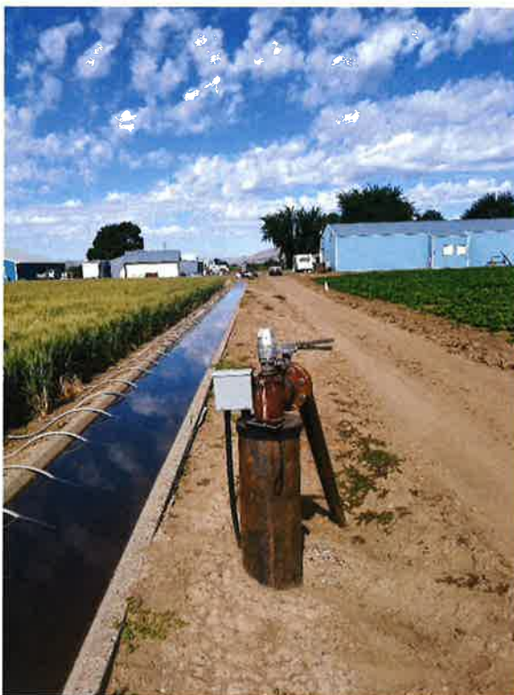
Well D0073175, looking west to the junction of the two mainlines.
