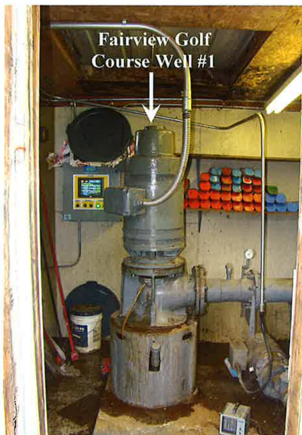
Photos of existing Fairview GC Well #1 pumphouse with flow meter that supplies water to irrigate the golf course.
