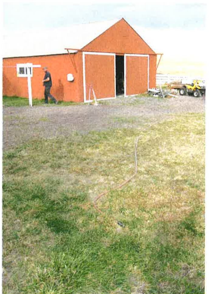
metal Shop BLDG flowing spigot
