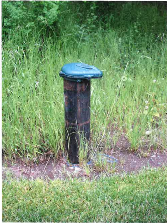
Figure 7: Injection Well (North Side of Home)
