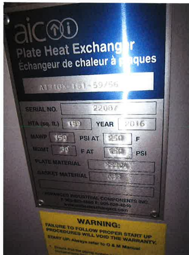
Figure 5: Heat Exchanger Tag
