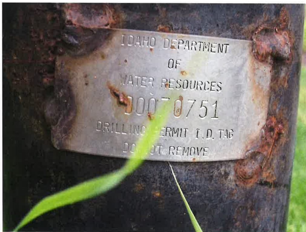
Figure 8: Tag on Injection Well
