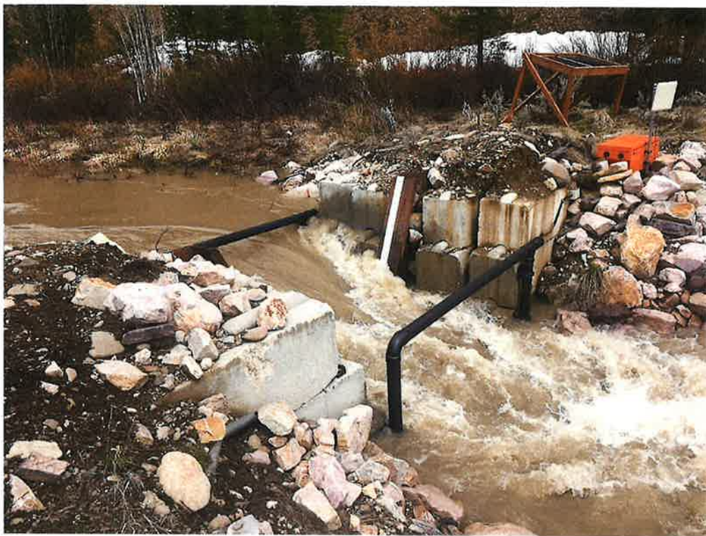
Attachment to 72-16896 Beneficial Use Field Report – Photographs from Trout Unlimited showing inlet structure under high flow conditions
