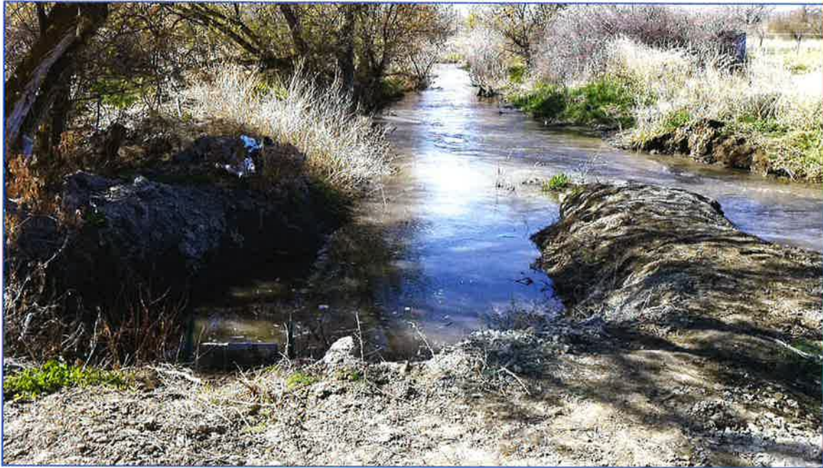
Figure 1: Point of diversion from Castle Creek. Diversion gate in left foreground.
