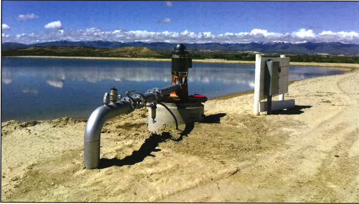
Figure 3: Irrigation storage reservoir south of Castle Creek Rd and 40-hp pump from pond to irrigation system north of Castle Creek Rd.
