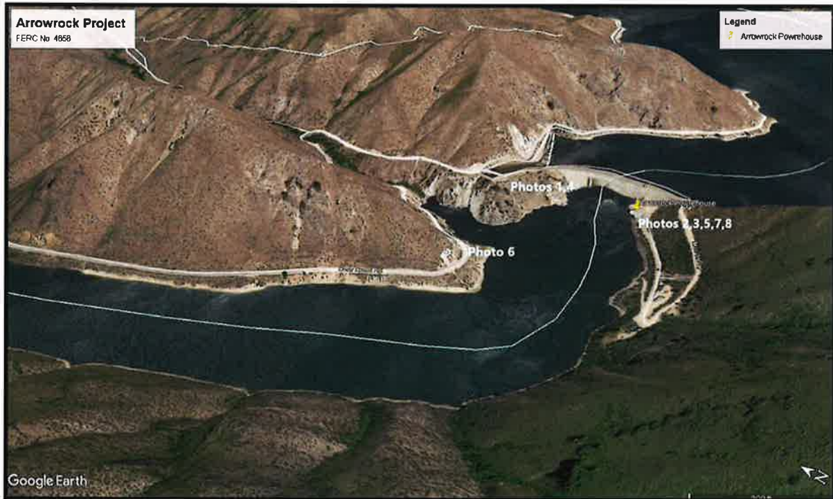
Figure 2. Photo location map of Arrowrock (FERC No. 4656) Hydroelectric Project.
