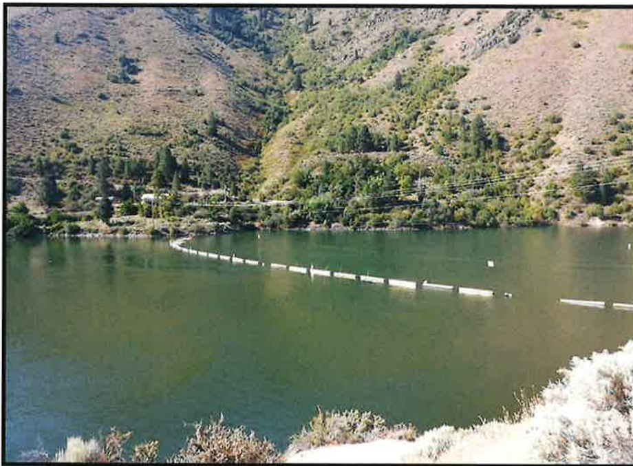
Photo 6. Boat barrier boom installed to prevent access to the dam.
