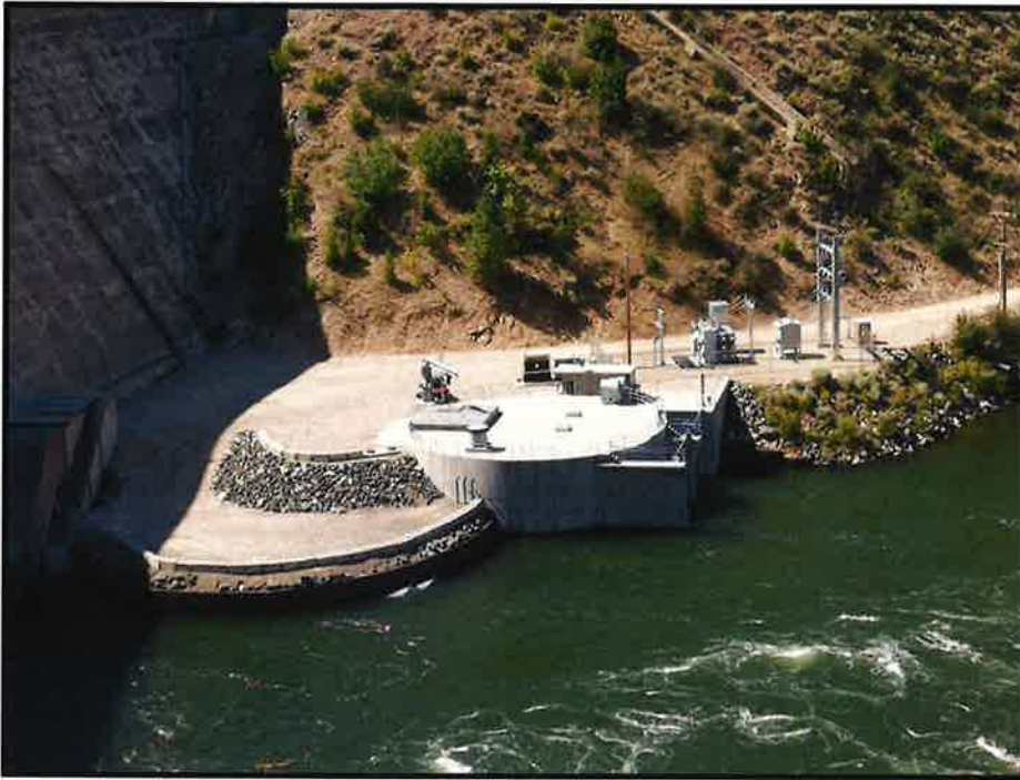
Photo 1. Arrowrock powerplant below dam.
