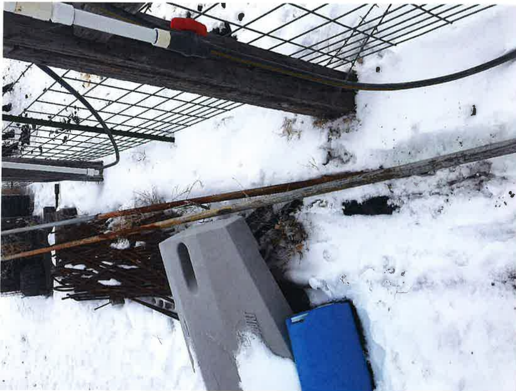
Figure 8. (con't) Pump and riser pipe recently removed from Schvaneveldt well.
