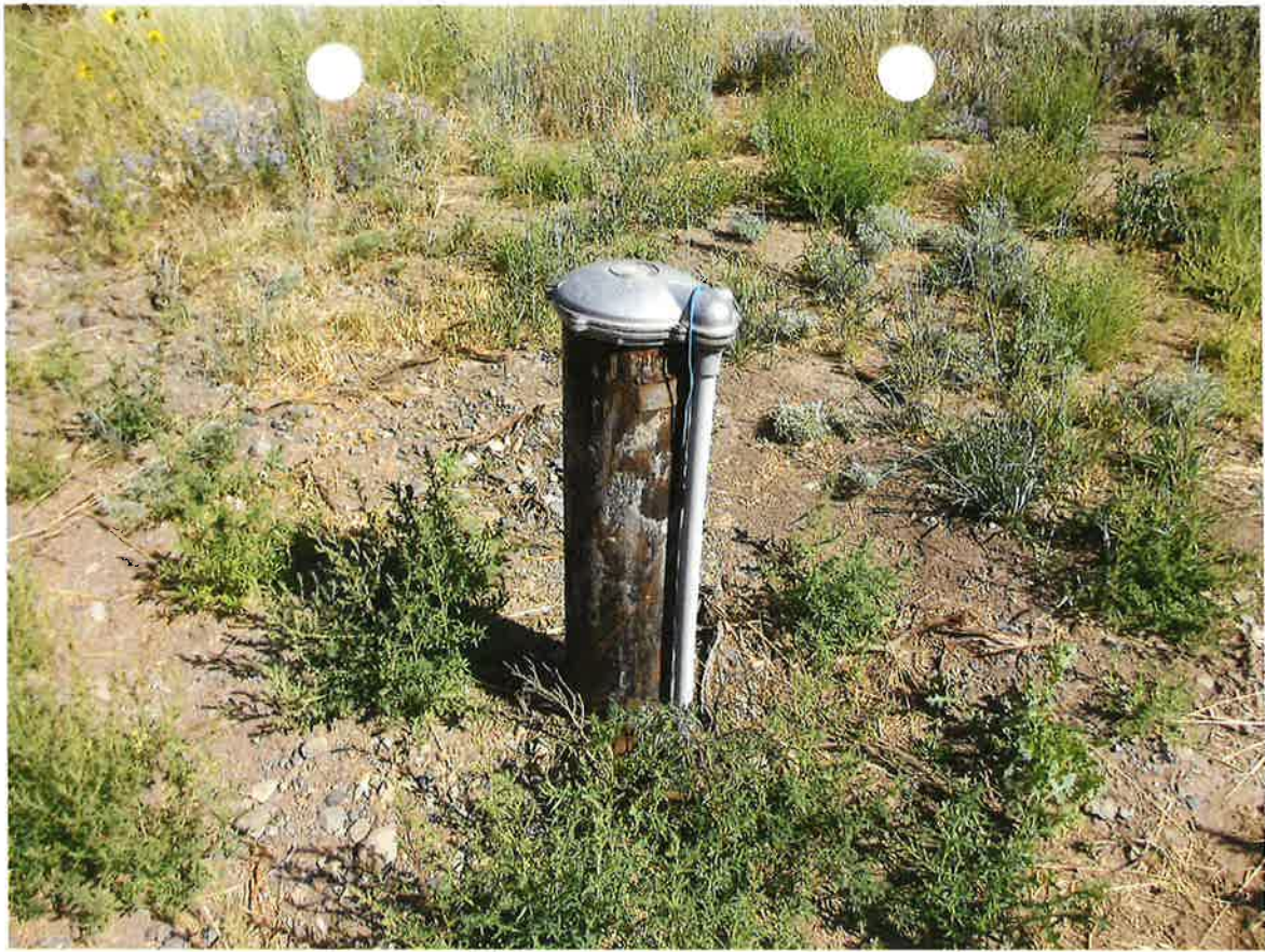
Point of Diversion
