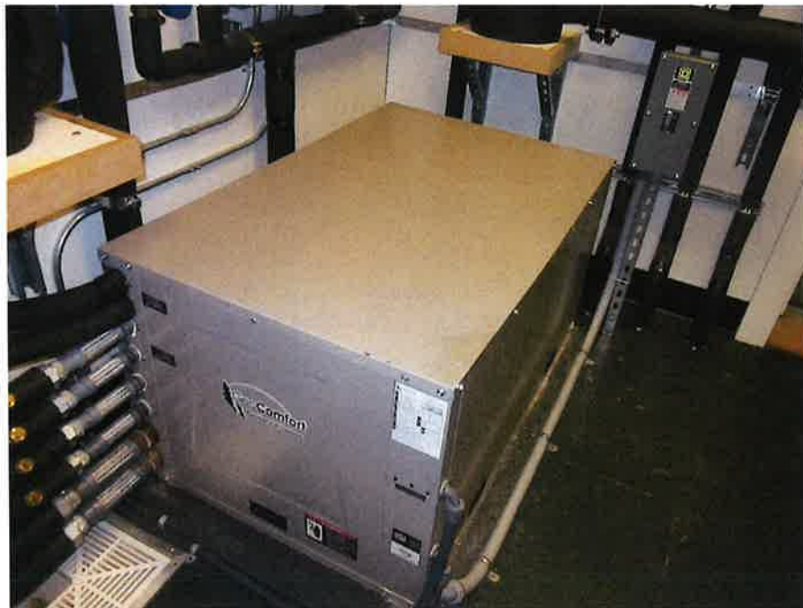
Figure 2: GeoComfort heat pump
