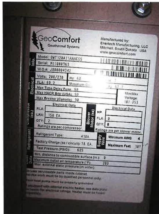
Figure 5: Tag on GeoComfort heat pump
