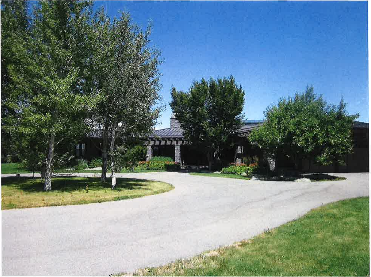
Figure 7: The Hagey residence (7,948 sf)
