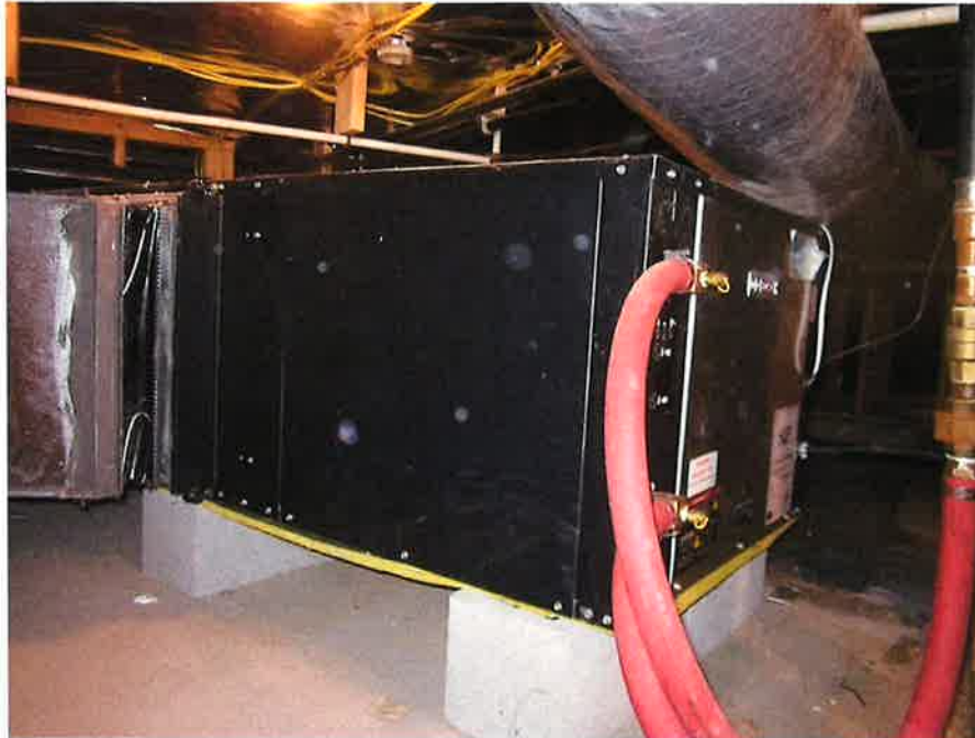
Figure 3: Bosch heat pump
