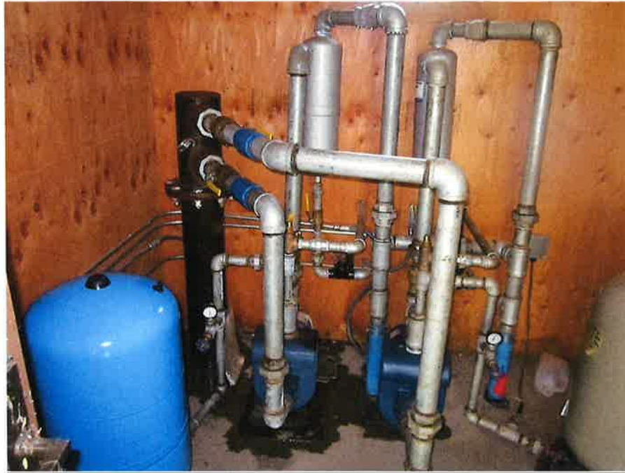
Figure 1: The well head in the pump house
