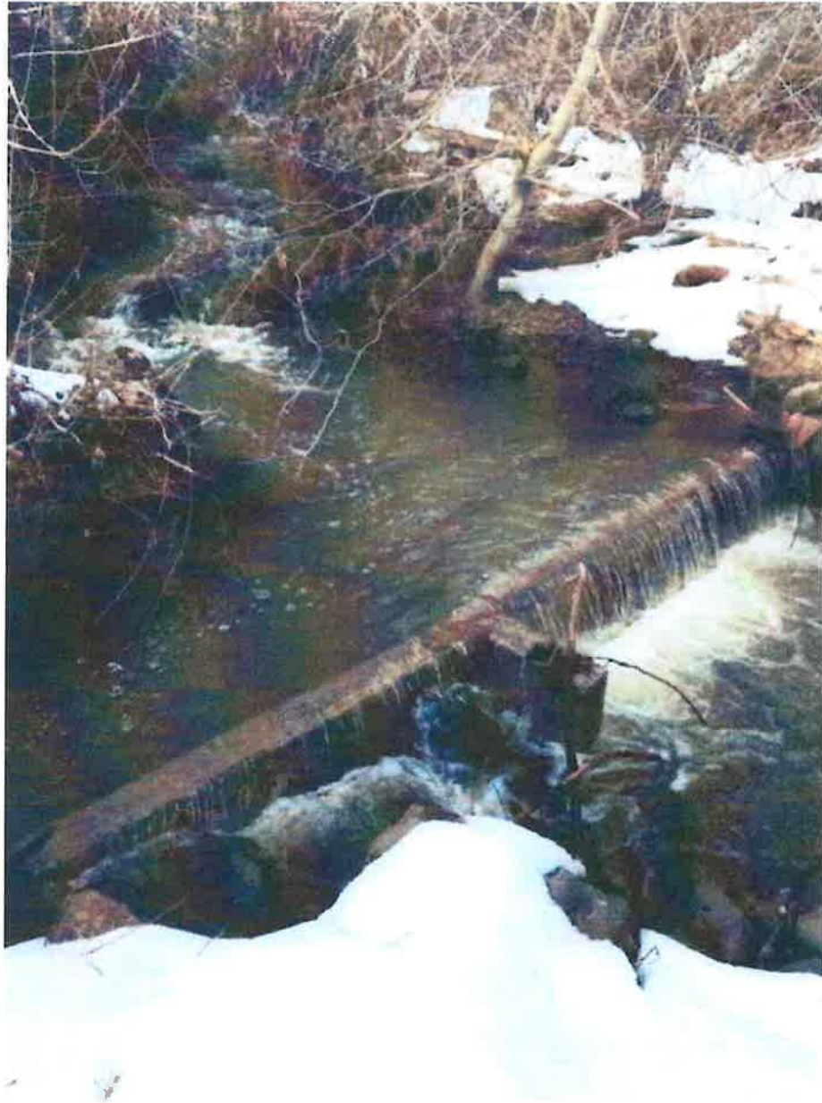
Jenkins Creek Reservoir Diversion 3-9-2019
