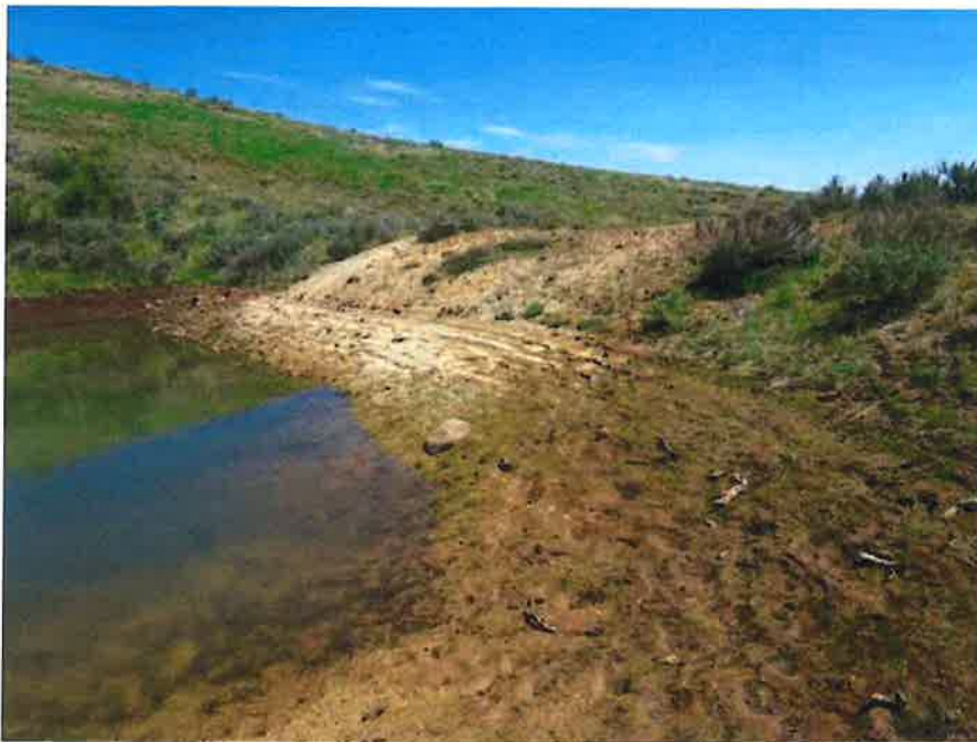
Photo 2: Pond No. 1 upstream slope of earthen embankment; note high water mark.
