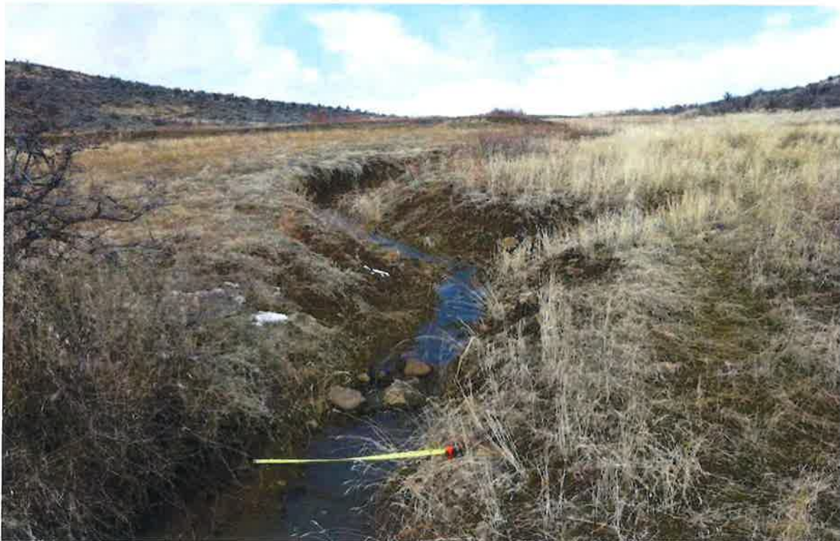
Photo 2: Pond No. 9 spillway channel; immediately downstream of impoundment.
