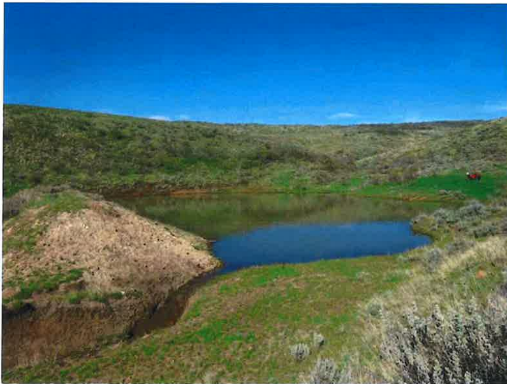
Photo 11: Pond No 4 spillway.
