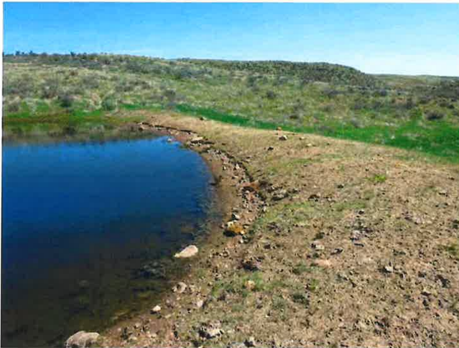
Photo 5: Pond No. 2 upstream slope of earthen embankment; note high water mark.
