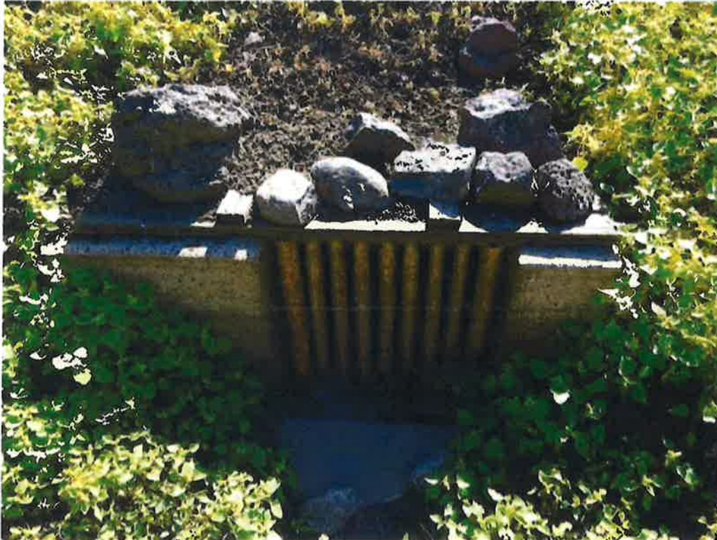
Photo 6: Inlet to outlet works; note free and clear of debris.
