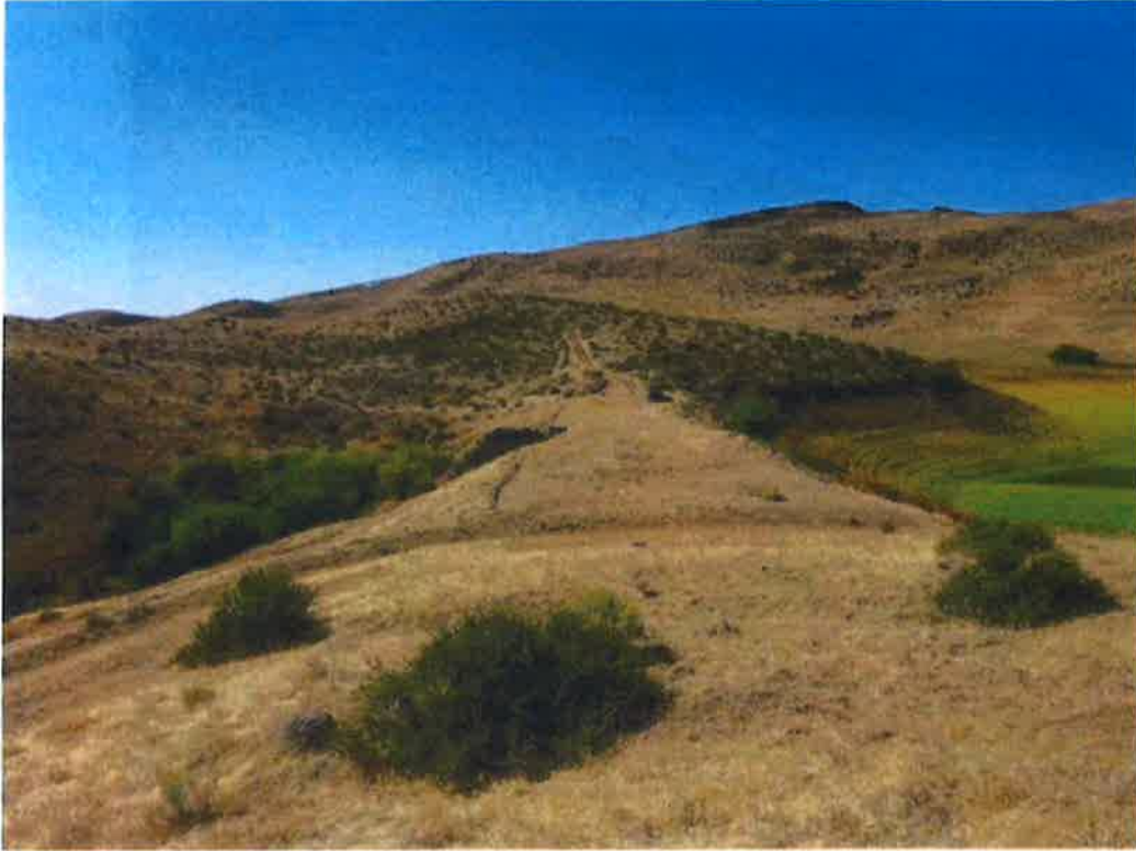
Photo 1: Jenkins Creek dam as viewed from above on the left abutment; note wide crest width.
