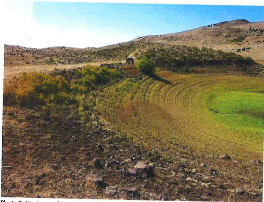
Photo 3: Upstream slope; note minor amount woody vegetation.
