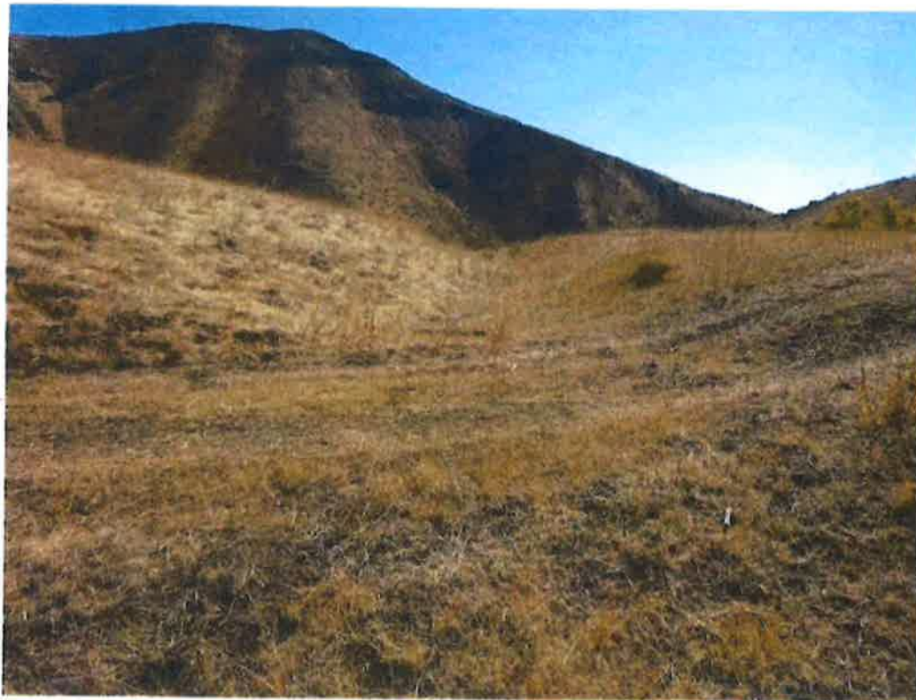
Photo 8: Open channel spillway located on left abutment.
