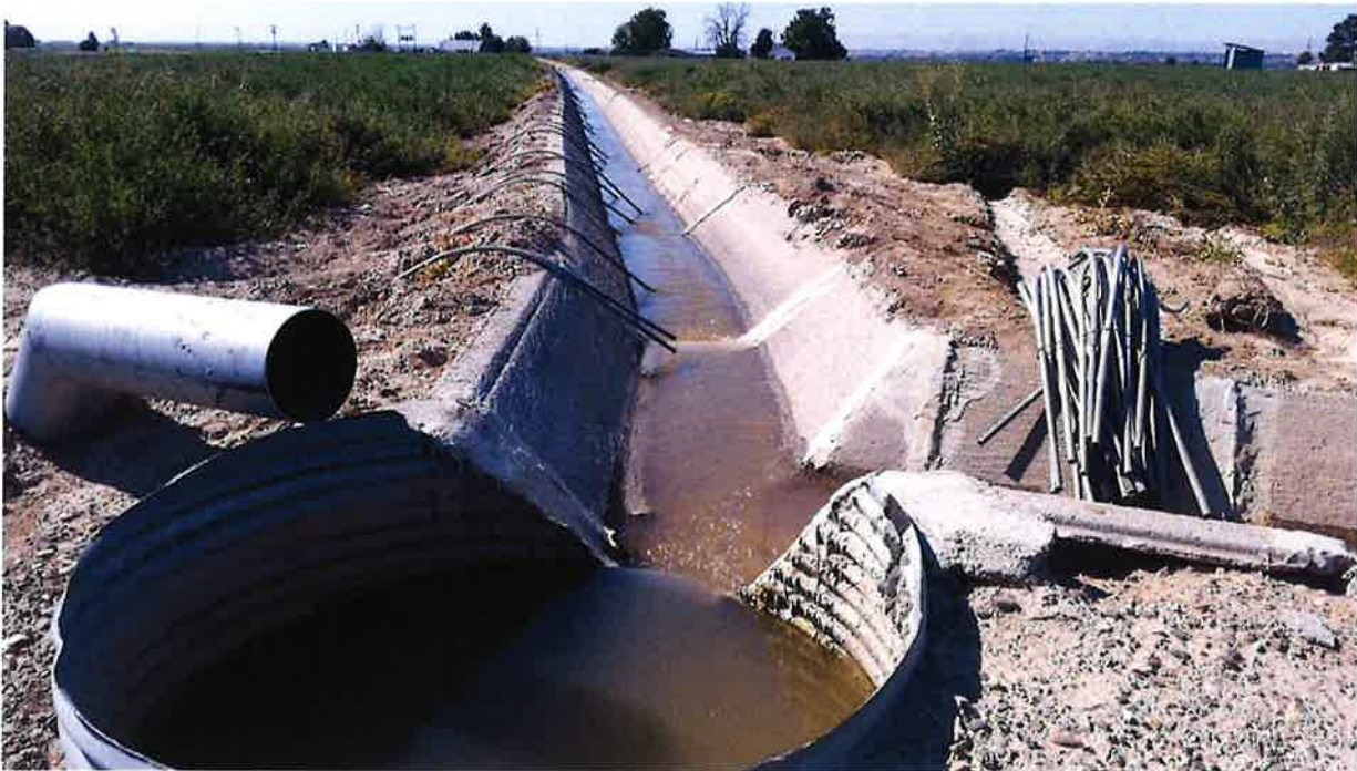
POD underground pipe to NW-SE and West trending ditches. Looking South.
