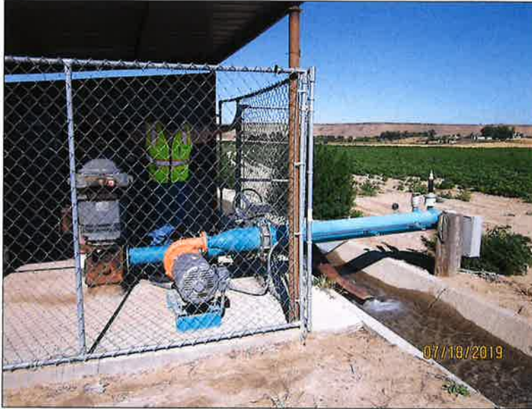
Figure 1: Looking west onto the POD, which is currently discharging into the open ditch.
