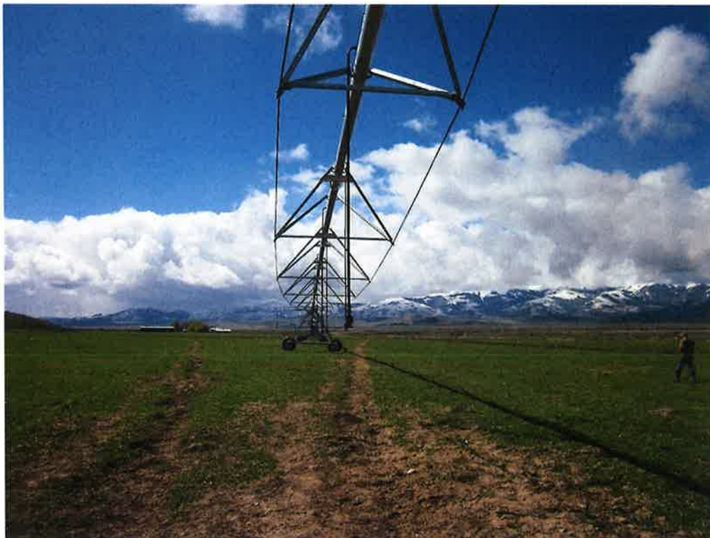
Figure 6: Looking south from center of new north pivot
