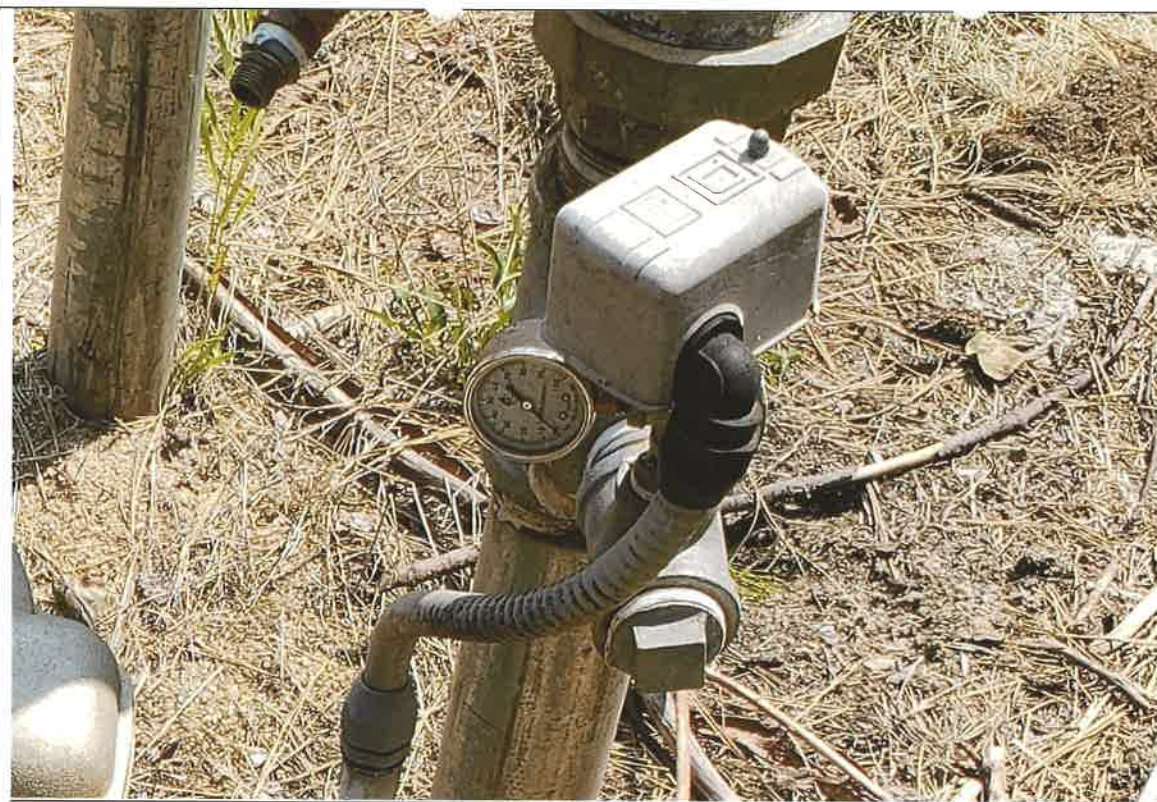
Figure 3. The pressure gage before the filtration system did not work and registered zero.
