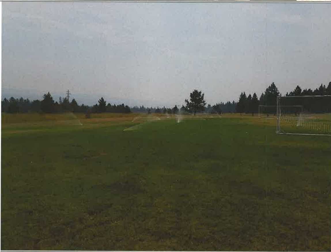
Figure 8. There were 11 separate irrigation zones with an average of 15 heads per zone. This photo shows the largest, zone 8, which runs 24 sprinkler heads.
