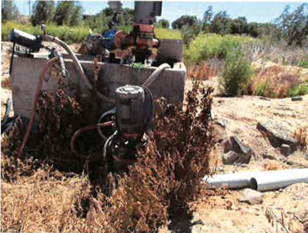
Artesian well for WR 63-31100 (no power hooked) up discharging into irrigation box Control valve between well and irrigation box 10" pipe running southerly discharging to Indian Creek located in T03NR01WS31 NESW
