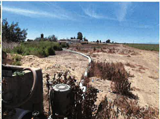
Artesian well for WR 63-31100 (no power hooked) up discharging into irrigation box Control valve between well and irrigation box 10" pipe running southerly discharging to Indian Creek located in T03NR01WS31 NESW
