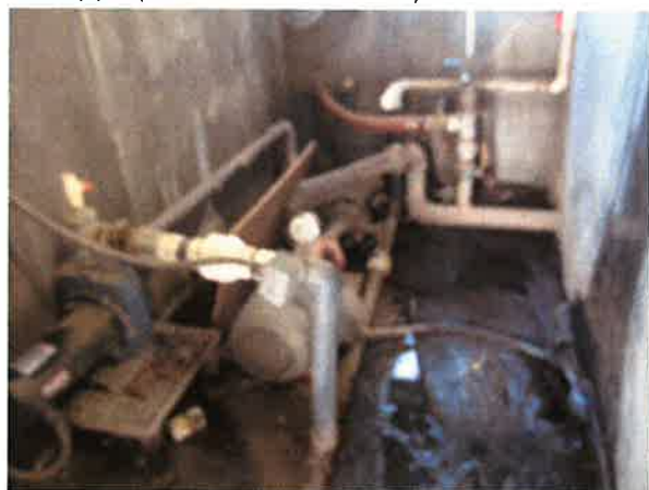
Inside of room next to re-use stock tank (130"X 204" X 120")
