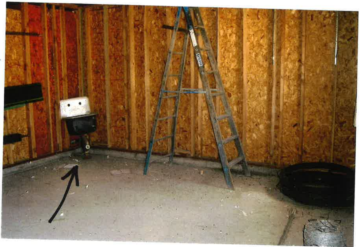
sink in building approximately 2004
