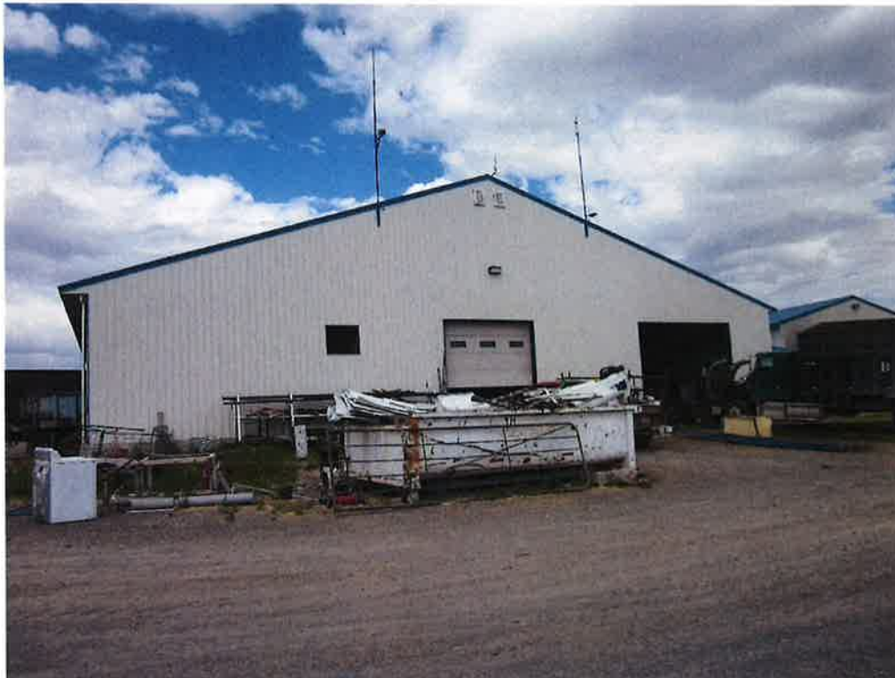
Figure 2: The shop addition
