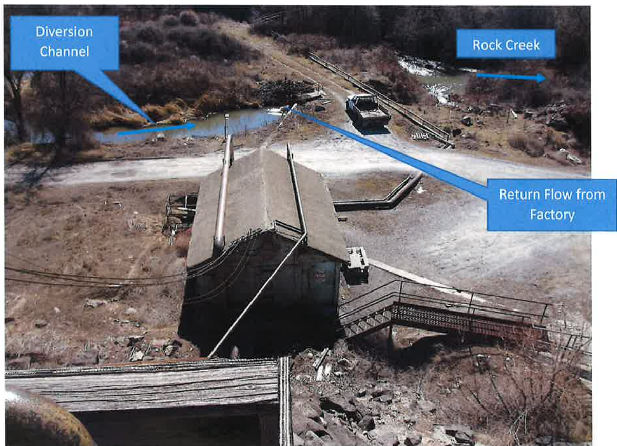
Overhead view of pump house and diversion channel
