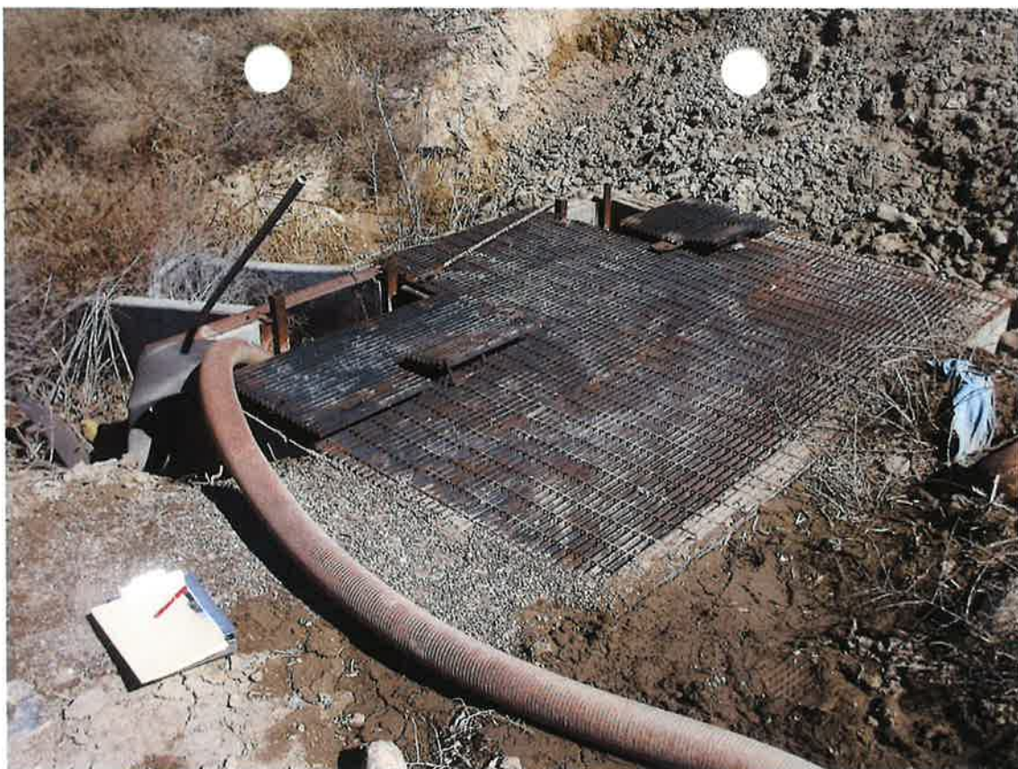
POD – Concrete collection box at drain tunnel
