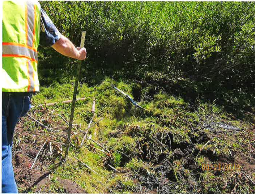
Figure 1. Point of diversion, buried spring box
