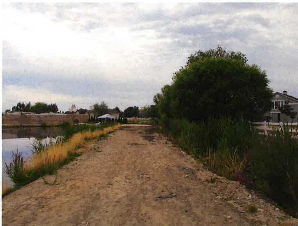
Photo 6 - Standing on the road showing the separation between the pond and the drainage canal.
