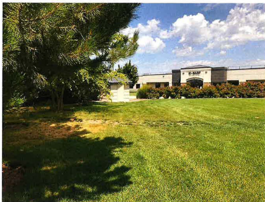
Photo #4 – Pump House and Irrigated Area
