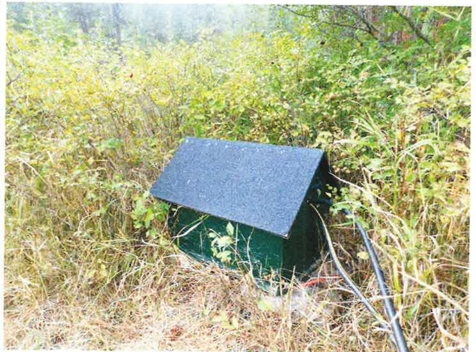
Pump House holding 1 hp Sprinkler Pump with timer drawing water from the Middlefork of the Payette. Distributes water via two hose pipes to above ground sprinklers per original application.
