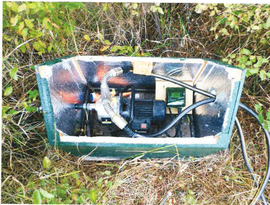
Pump House holding 1 hp Sprinkler Pump with timer drawing water from the Middlefork of the Payette. Distributes water via two hose pipes to above ground sprinklers per original application.
