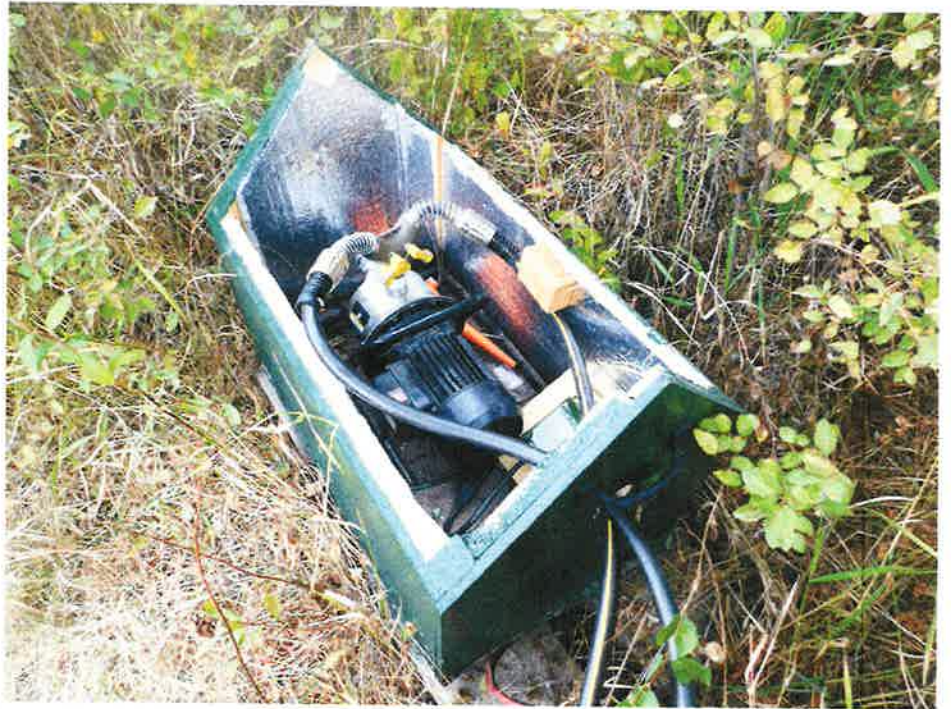
Pump House holding 1 hp Sprinkler Pump with timer drawing water from the Middlefork of the Payette. Distributes water via two hose pipes to above ground sprinklers per original application.
