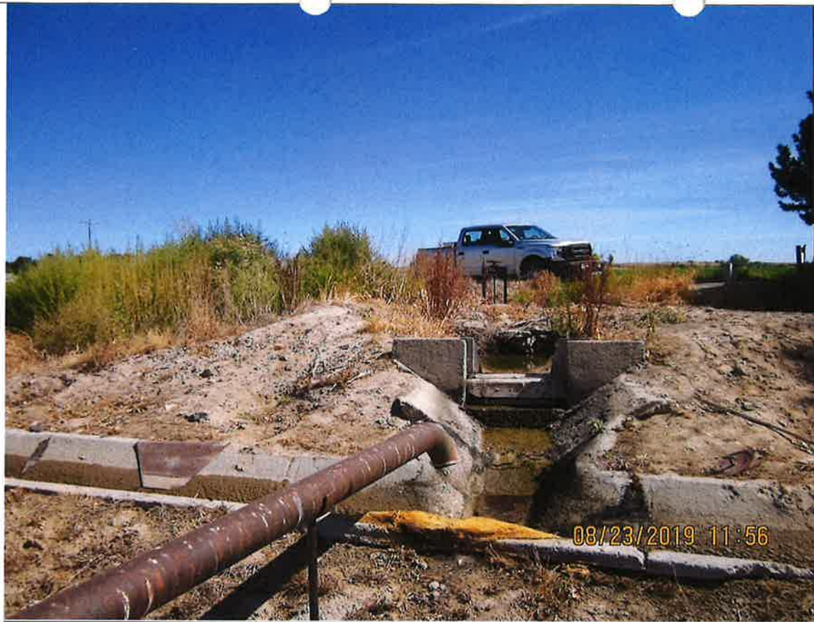
Figure 7. Source of surface water through black metal headgate labeled 2.46.
