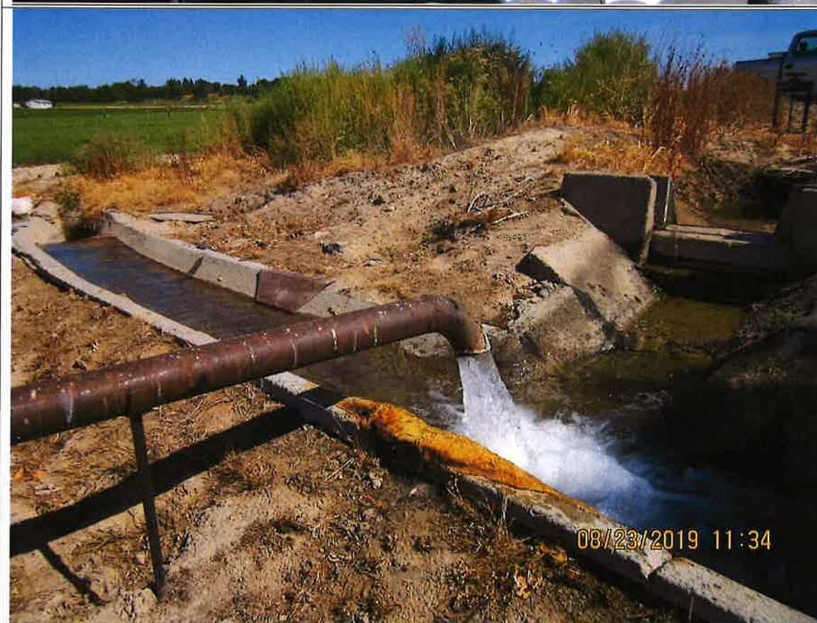
Figure 4. Open discharge from well into concrete ditch.
