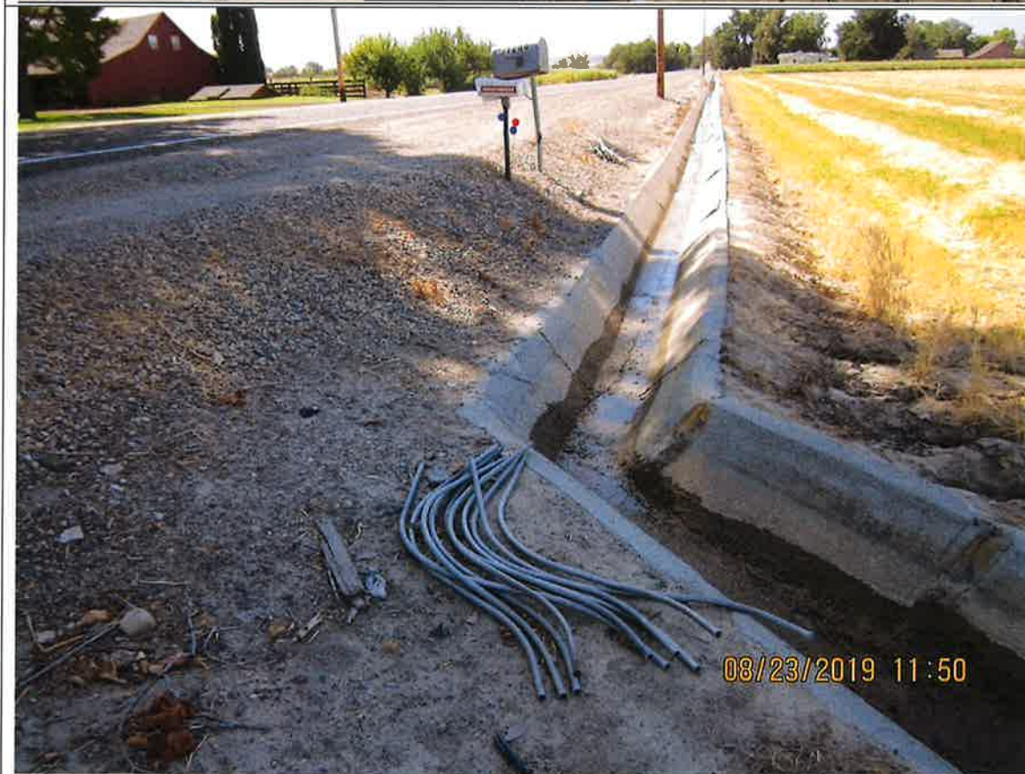
Figure 6. Surface water is delivered to field via a concrete ditch and siphon tubes.
