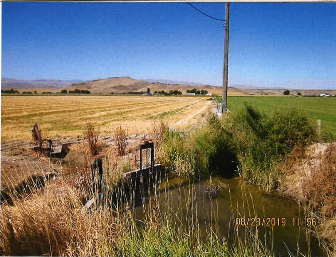
Figure 8. Surface water being diverted into pipeline and conveyed to ditch in the center of the field.
