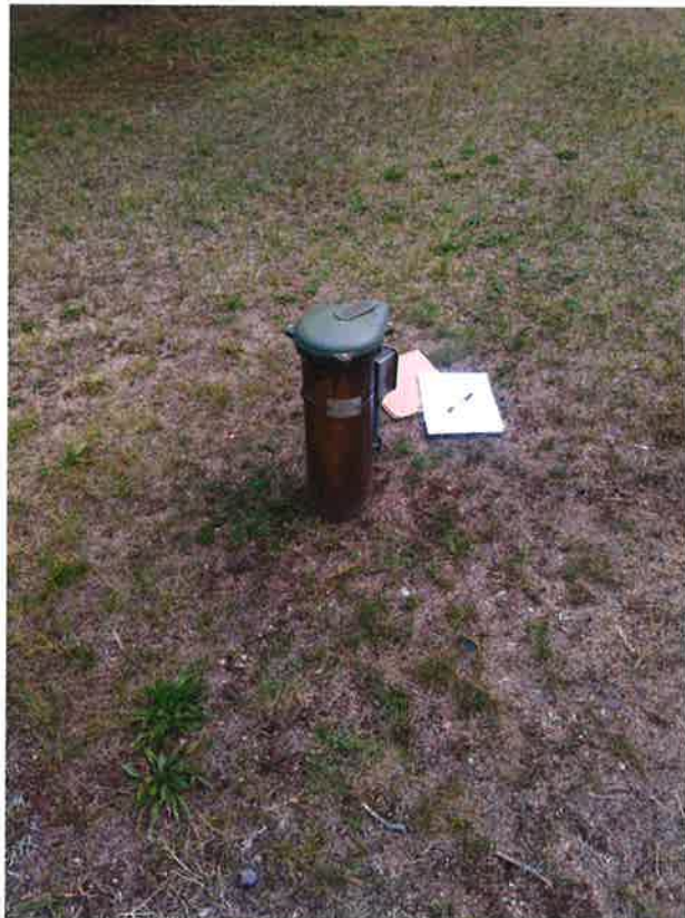
The six-inch well used as the point of diversion for this right.
