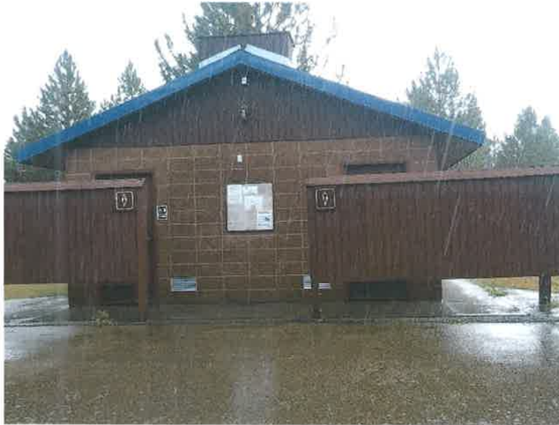
The bathroom unit for the campground.
